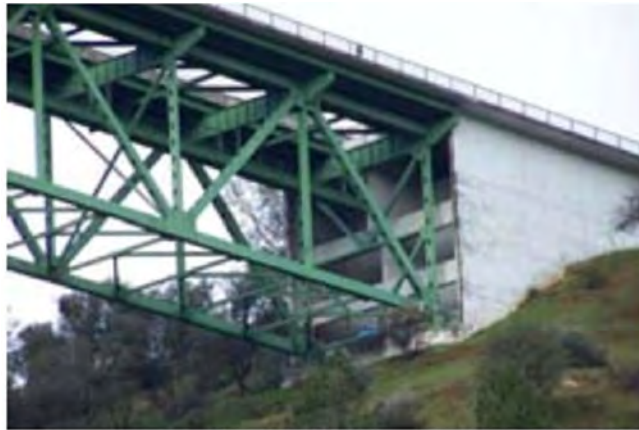
Figure A-23 Abutment of the Bridge
