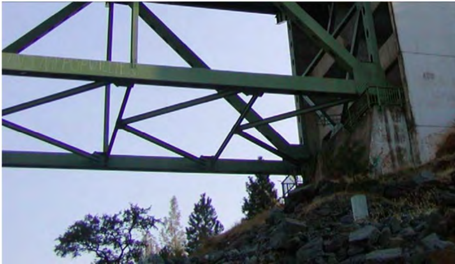
Figure A-26 Lower Horizontal Bracing Near Abutment
