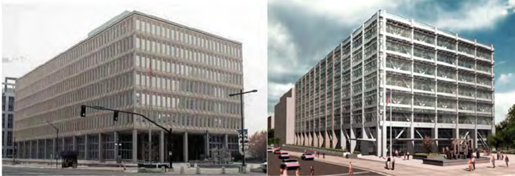
Figure A-11 Wallace F. Bennett Building Prior and Post Rehabilitation (Aiken et al., 2001)
