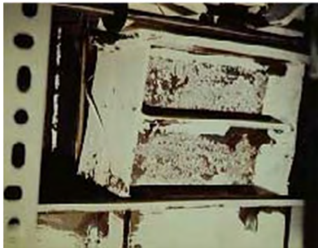
Figure A-42 Deflected Shear Links and Visible Buckling in the Flanges (Zahrai and Bruneau, 2000)
