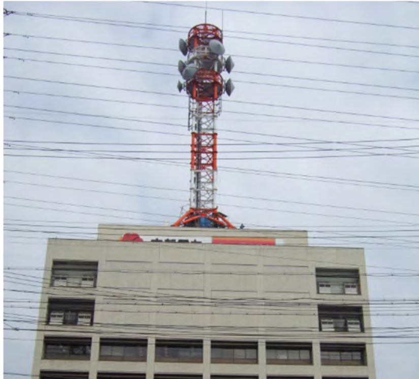
Figure A-30 A Telecommunication Tower in Japan (Courtesy of Ian Aiken, Seismic Isolation Engineering, Emeryville, California)
