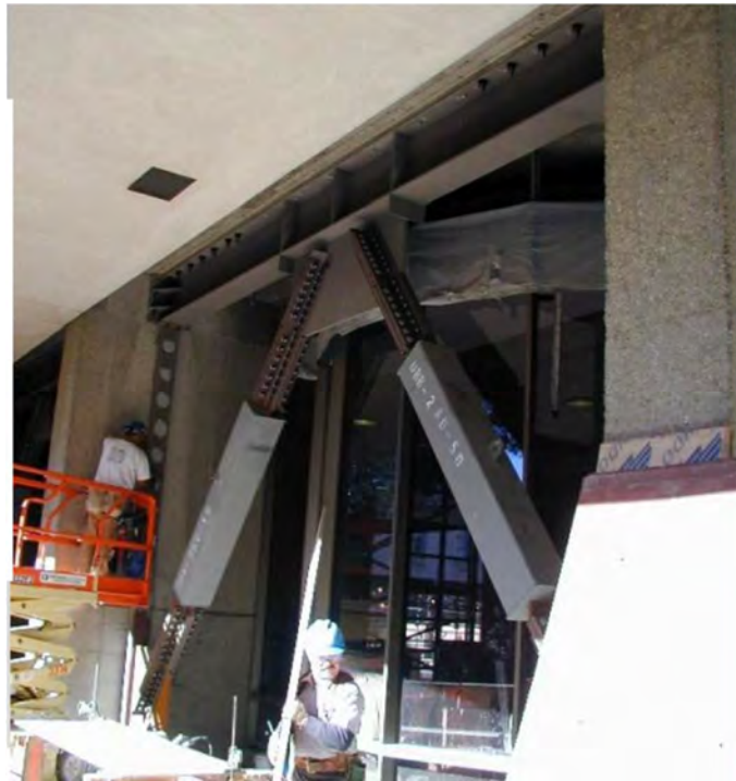
Figure A-15 BRB Connection Details (Anagnos T., 2011)
