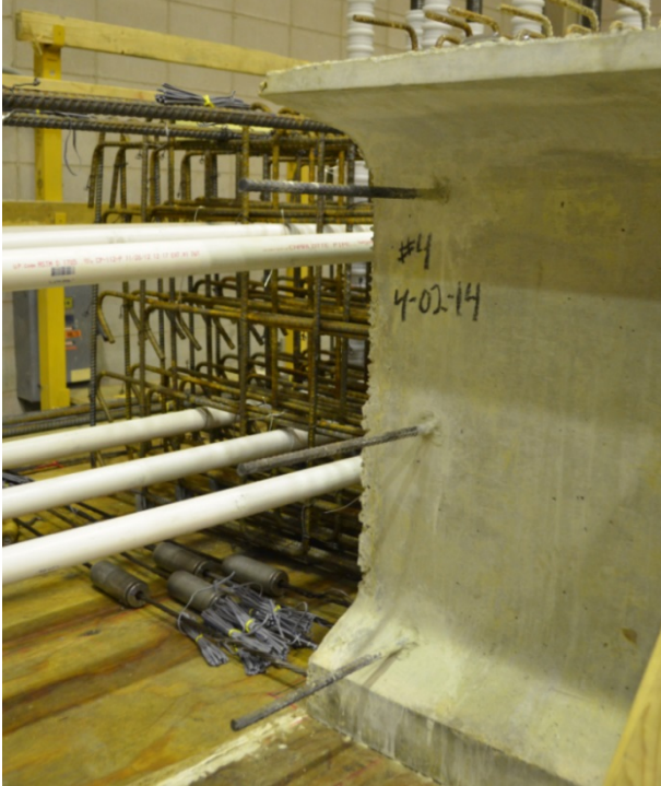
Figure 5.6: Dowel bars inserted through the web of girder
