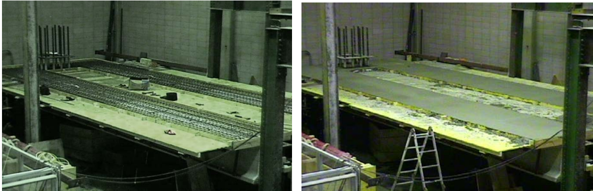
Figure 4.16: Individual bridge decks before (left) and after (right) concrete pour
