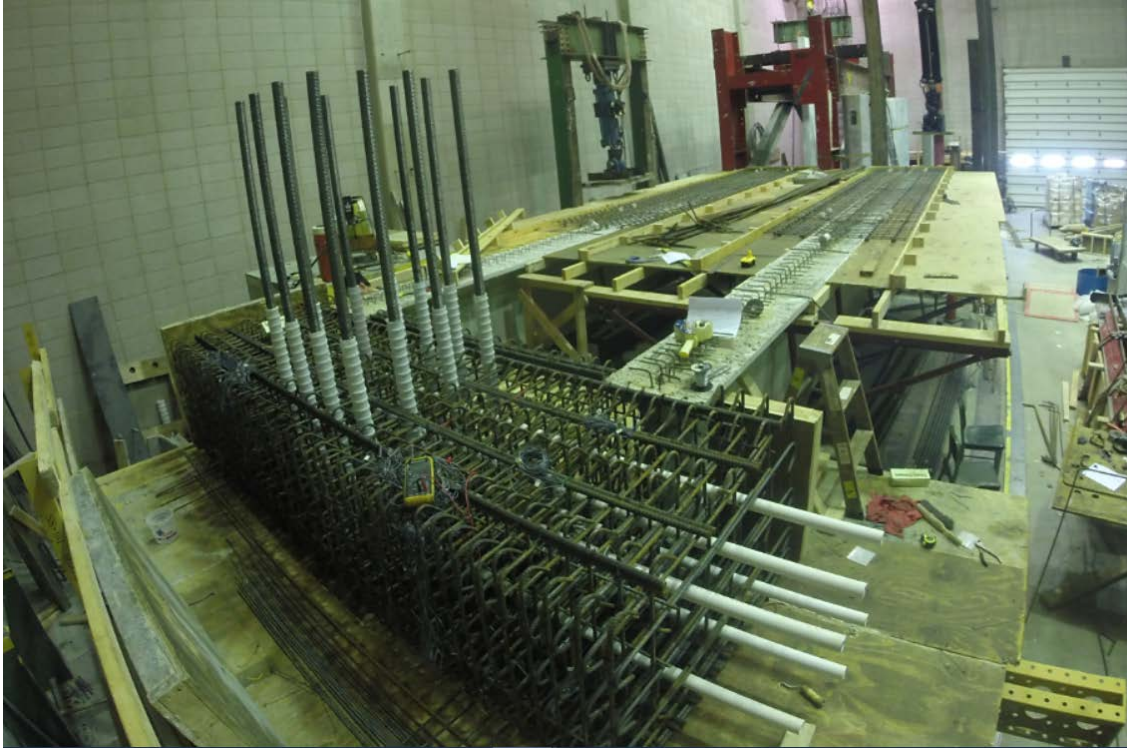
Figure 5.8: Reinforcement cage for bent cap and deck reinforcement
