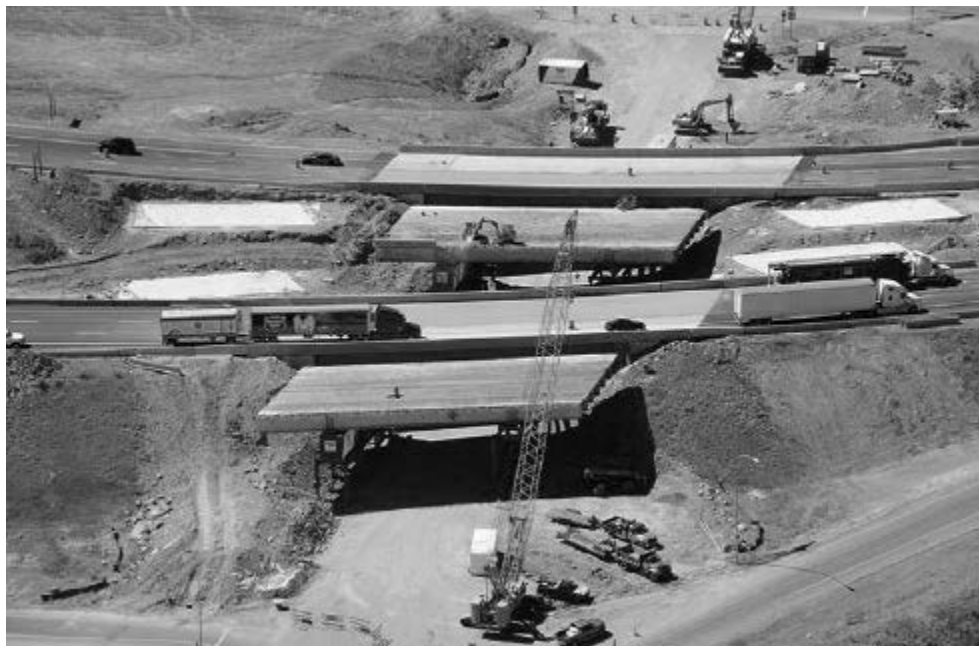
Figure 1.2: Lambs Canyon Bridge constructed using ABC methods (FHWA, 2010)
