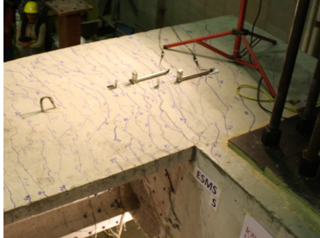
Figure 5.21: Flexural cracks formed on the deck of the ESMS Connection
