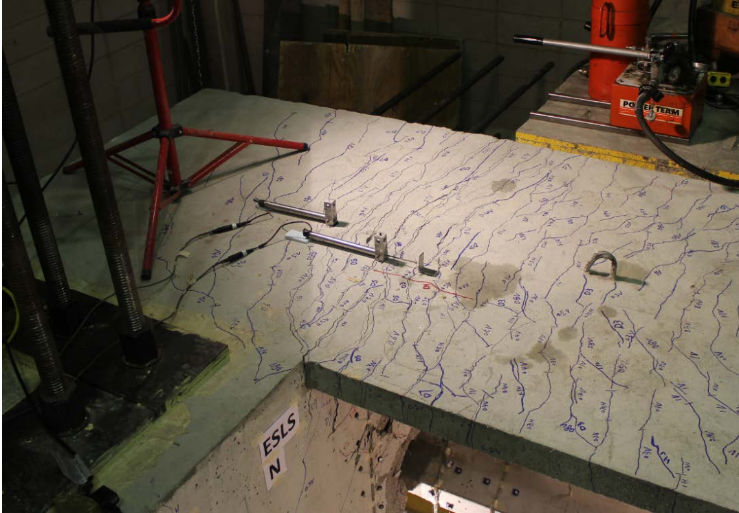
Figure 5.29 Cracks on Deck of the ESLS Connection
