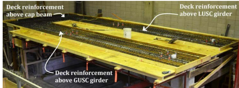
c. Deck formwork and reinforcement
