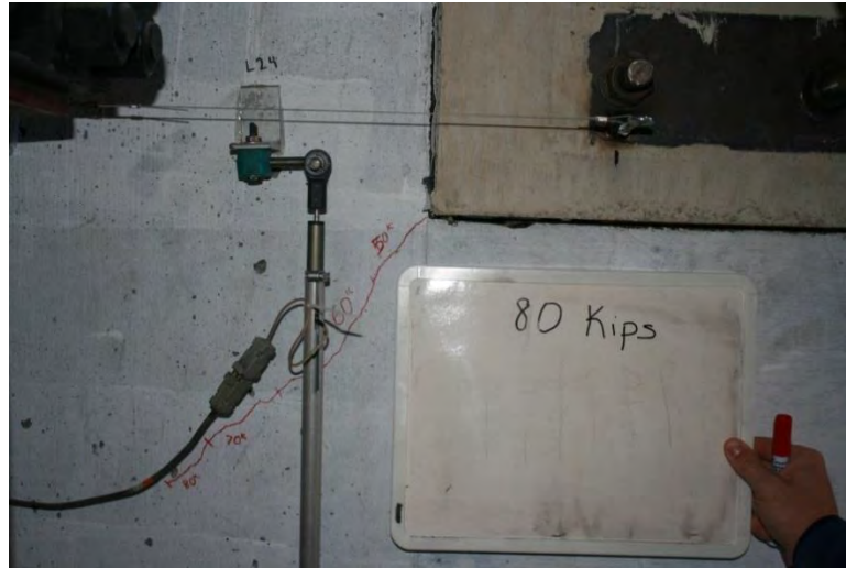
Figure 6.45 Propagation of first diagonal crack on the east face of shear key 8B
