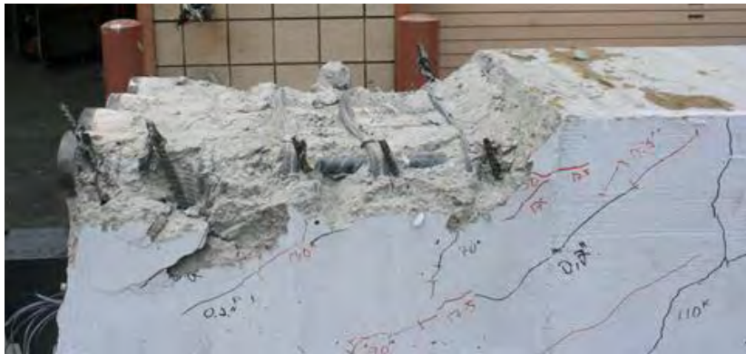
Figure 6.92 Sliding surface after removing shear key 10A
