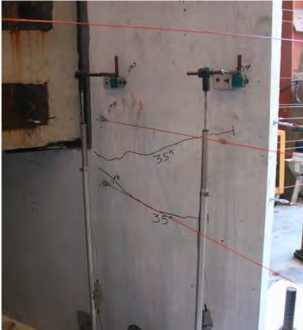
Figure 8.30 First cracks observed on the southeast side of shear key 12B
