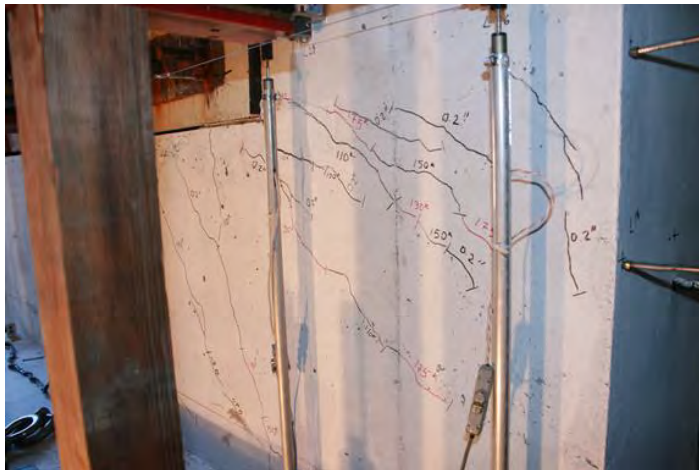
Figure 6.73 Cracks on the west face of shear key 9B at a displacement of 0.20 in.
