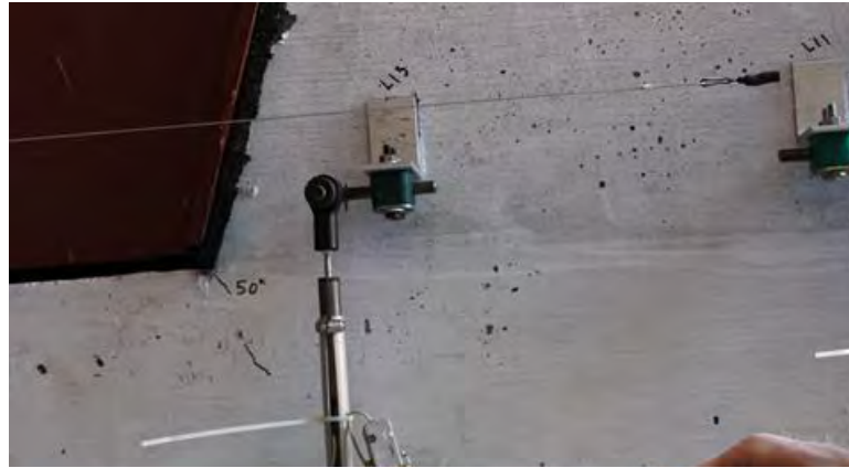
Figure 6.29 First diagonal crack observed on the east face of shear key 8A
