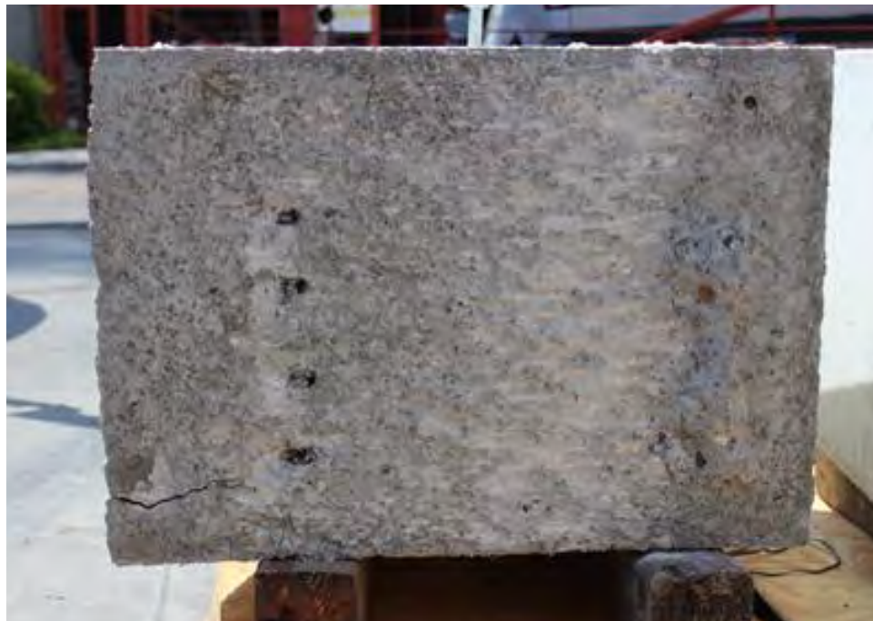
Figure 5.41 Sliding plane condition for shear key 7B after the completion of the test
