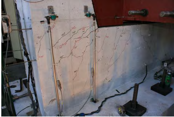
Figure 6.59 Cracks on the west face of shear key 9A at 210 kips
