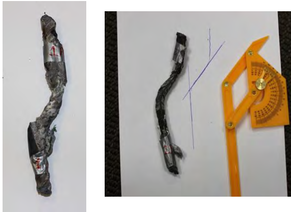
Figure 5.28 Extracted dowel bars from shear key 7A showing the angle of inclination
