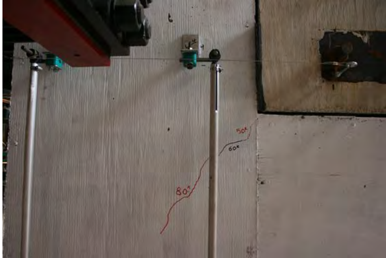
Figure 6.100 First crack observed on the east face of shear key 10B
