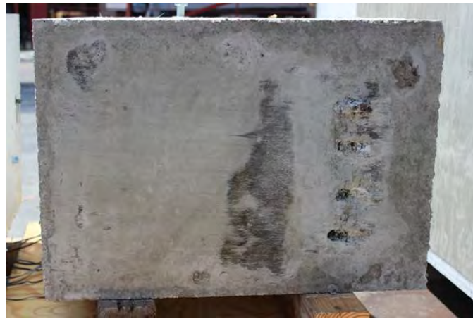
Figure 5.29 Sliding plane condition for shear key 7A after the completion of the test
