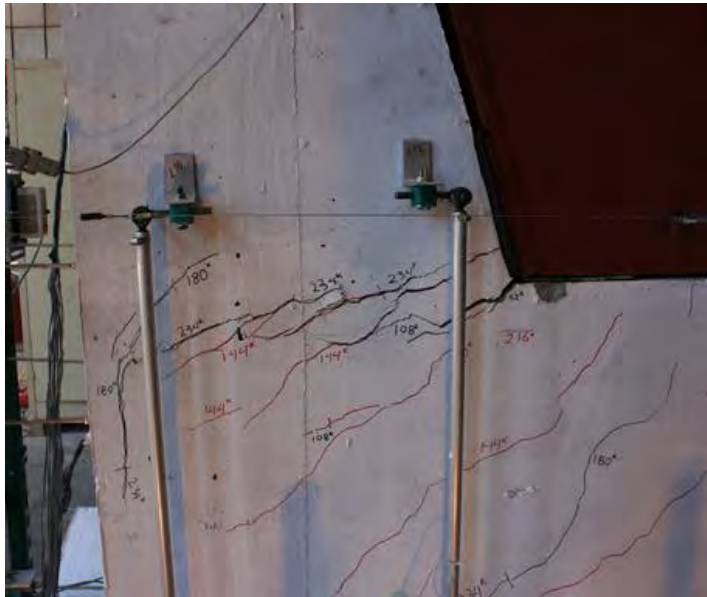
Figure 6.89 Diagonal cracks join to form a sliding plane on the west face of shear key 10A
