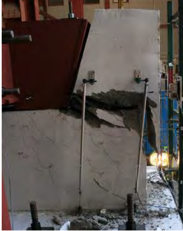
Figure 6.90 Sliding shear plane from the east face of shear key 10A
