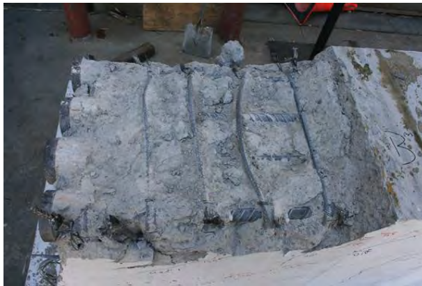
Figure 6.63 Sliding plane condition after shear key 9A was removed
