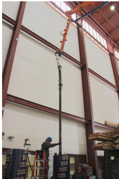
Figure 2.12 – Concrete placement using pump-fed tremie
