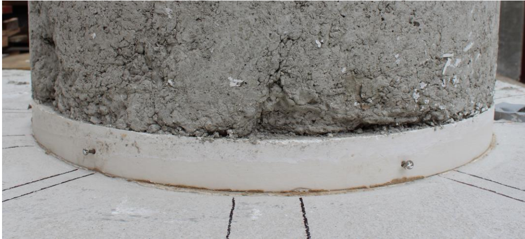
Figure 3.23 – Bottom of Pile Specimen #11 showing gaps
