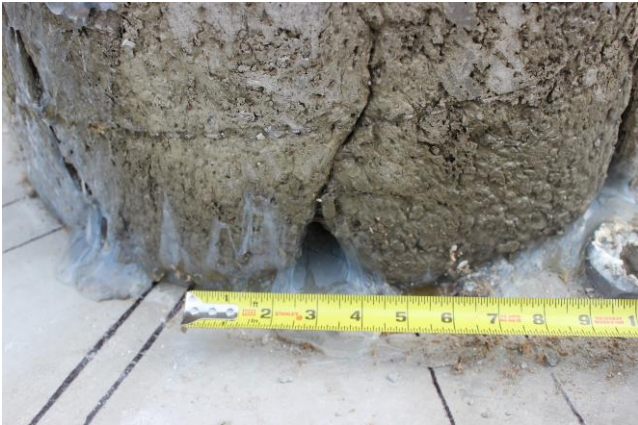
Figure 3.11 – Bottom of Pile Specimen #5 showing void at base
