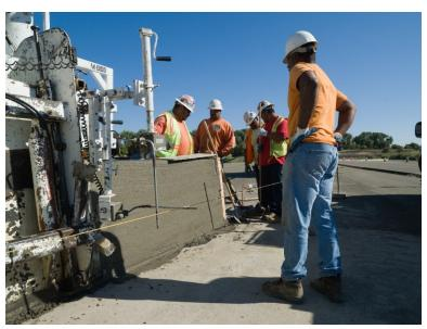
Figure 2-4 Slip-forming the Barrier
