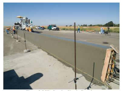
Figure 2-5 Slip-forming Nearly Complete
