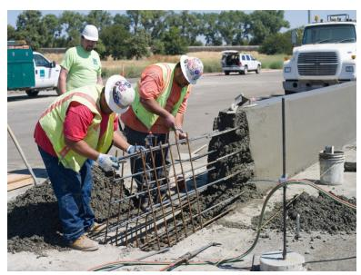
Figure 2-6 Placing Rebar for the End Anchorage
