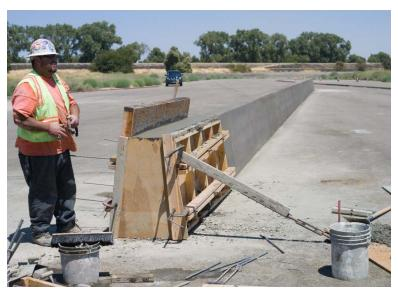
Figure 2-8 End Anchorage Pour Complete
