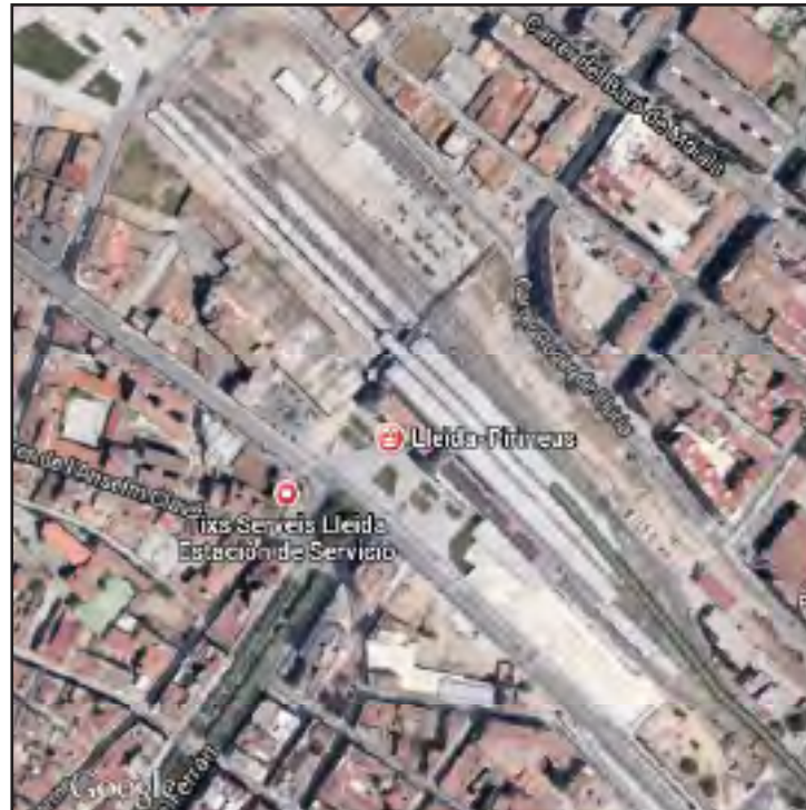
Figure 92. Aerial View of Lleida-Pirineus Station
