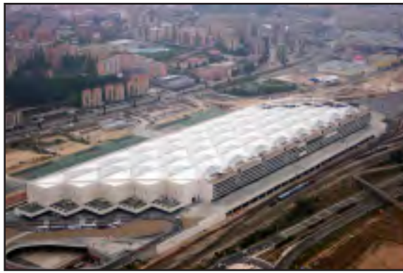
Figure 76. Exterior of Delicias Station
