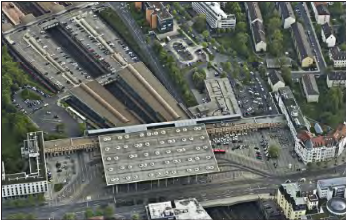
Figure 46. Aerial Close Up of Kassel Wilhelmshöhe
