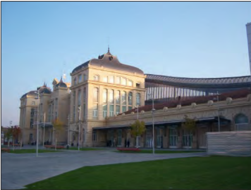
Figure 94. Façade of Lleida's Historic Railway Station
