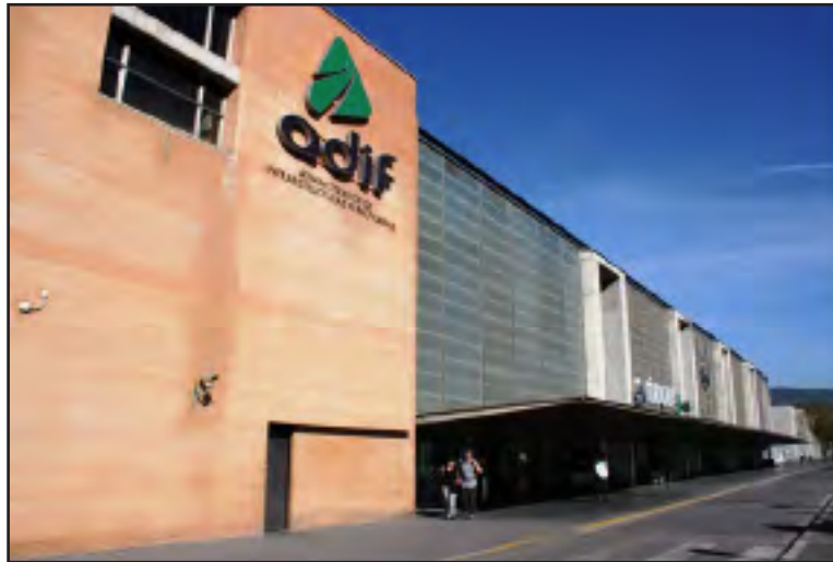
Figure 90. Façade of Córdoba Central Station
