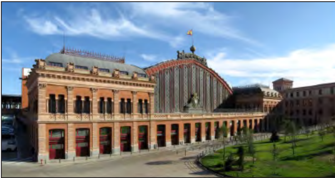
Figure 62. Façade of the Historic Atocha Station
