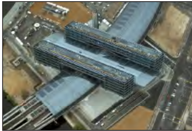
Figure 30. Aerial View of Berlin Central Station at Opening (2006)
