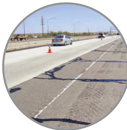
Results of a Sealzall manual sealing operation on Interstate 8 in Winterhaven
