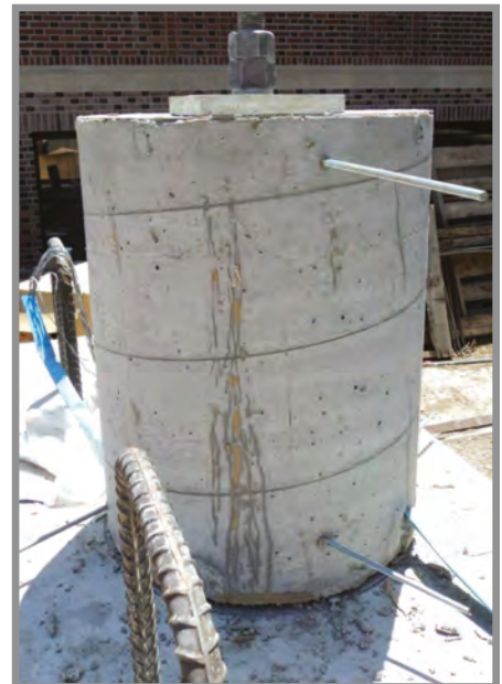
Pedestal with pipe pin connection at base
