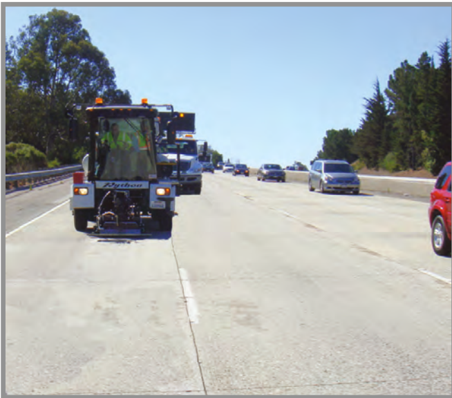
Python automated hot asphalt patching
