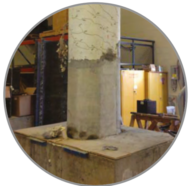
R-Calt-1 after concrete repair
