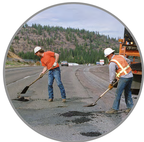
Manual pothole patching
