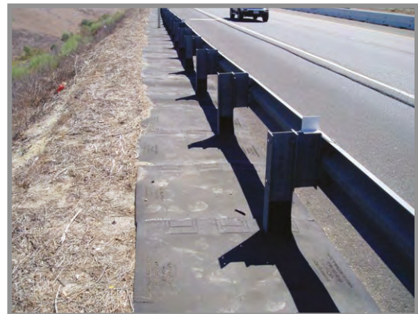
The redesigned guardrail is engineered for today's higher passenger vehicles.
