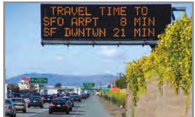
Posted travel times on changeable message signs is popular with the traveling public.
