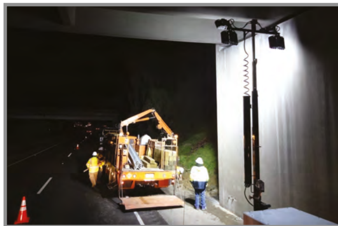
Night guard rail repair
