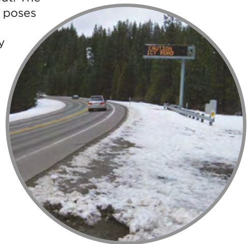
A changeable message sign activated by the ASWSC
