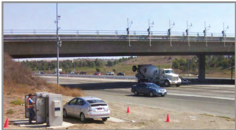
V2DVS equipment cabinets with pole-mounted vehicle detectors and bridge-mounted cameras and vehicle detectors
