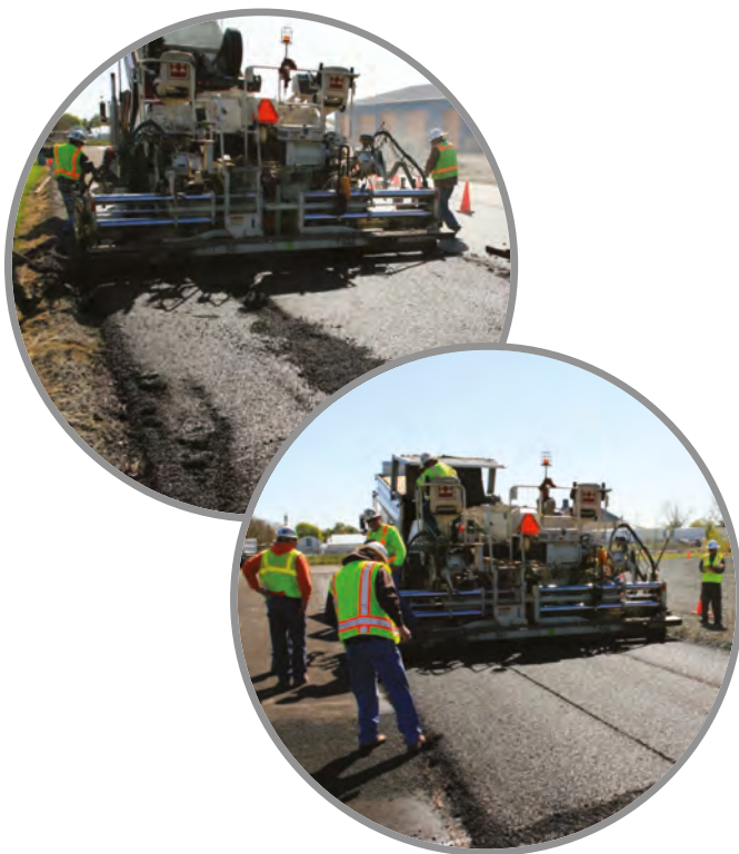
Paving with RHMA (left); working with RWMA (right)
