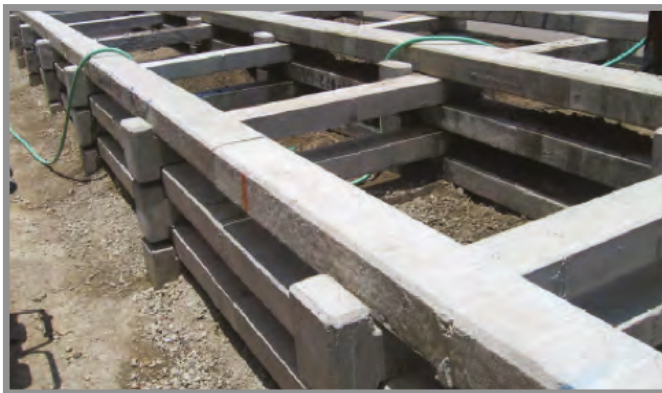
Precast concrete crib walls
