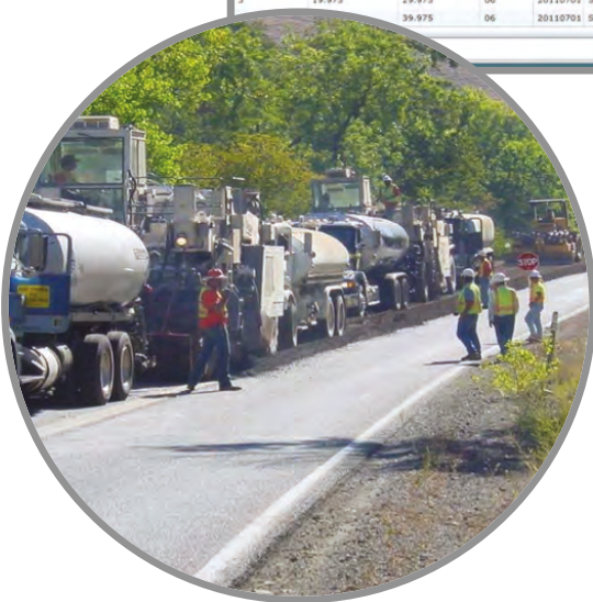
Foamed asphalt recycling project
