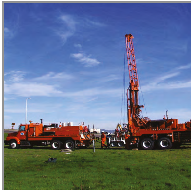
Drilling a downhole array at the Napa River bridge
