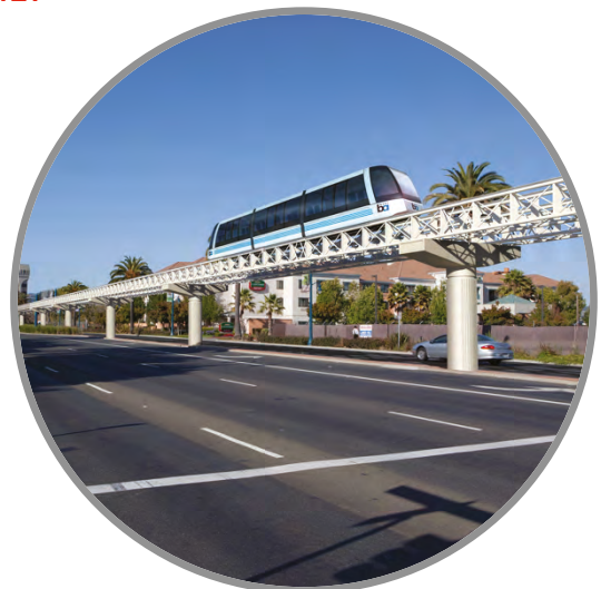
Oakland Airport Connector— an automated people-mover link from the BART Coliseum/ Oakland Airport station Source: bart.gov
