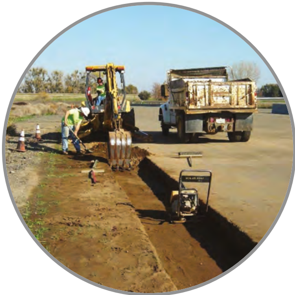
Excavation for barrier installation
