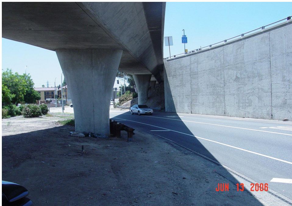
Madre St On-ramp – Looking West
