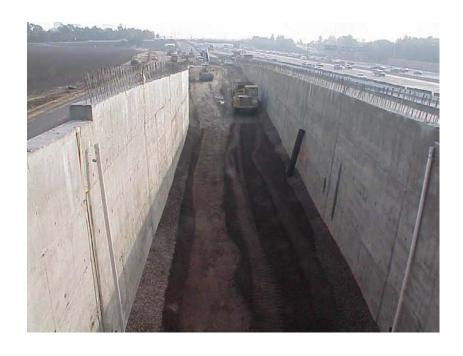
Figure 3.3.21 Backfilling at Abutment 1
