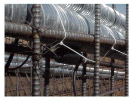
(a) LVDT Type Strain Meter Installed in the Deck
