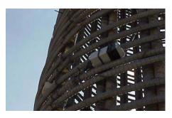
Figure 3.3.19 Installation of Signal Box for Conventional Strain Gauges
