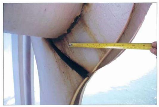
Fig. 3 Location of cracked eye bar.
