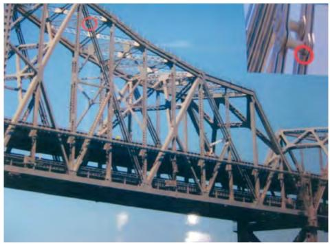
Figure 1: San Francisco-Oakland Bay Bridge East Span. Circled area is location of failed eye bar.
