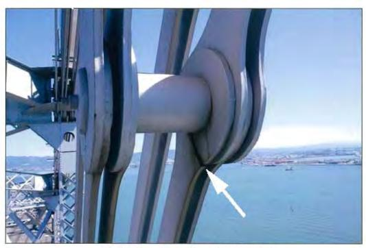
Fig. 2 Location of cracked eye bar. (Looking East)
