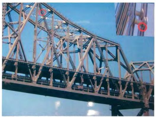
Fig. 1 San Francisco-Oakland Bay Bridge East Span. Location of cracked eye bar.
