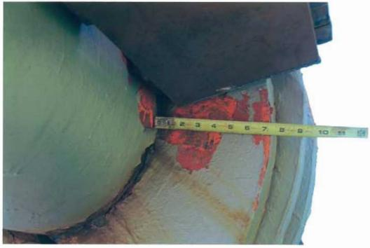
Fig. 6 Eye bar above crack location.
