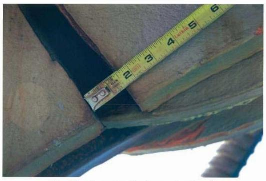
Fig. 8 Crack opening displacement, outer edge.
