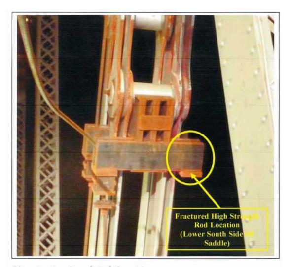
Fig. A Fractured Rod location.
