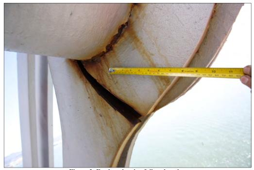
Figure 2: Eye bar showing failure location
