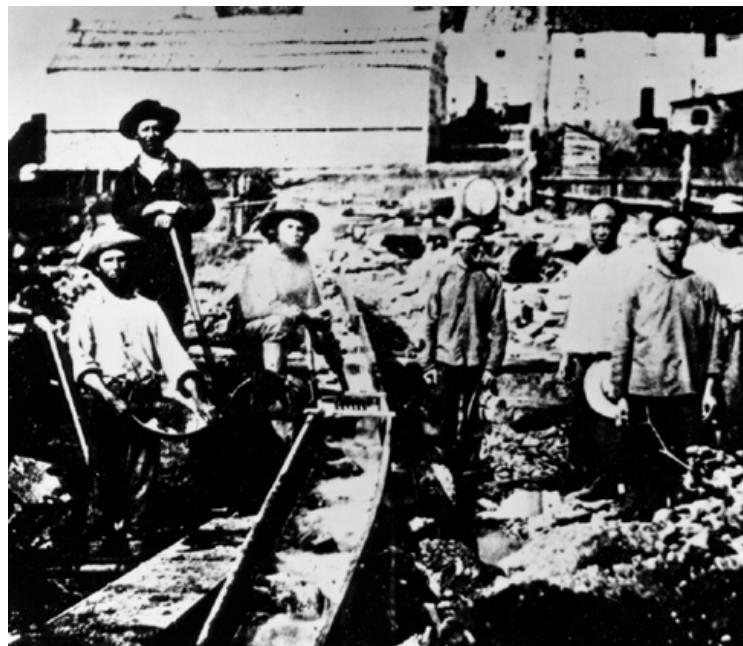
Figure 36. Chinese and White Miners Sluicing at Auburn Ravine, Placer County, ca. 1852 (used with permission, California Department of Conservation, California Geological Survey).
