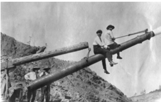
Figure 26: Men Astride Giants (monitors) at the La Grange Mine, Trinity County, n.d. (used with permission, California Department of Conservation, California Geological Survey).
