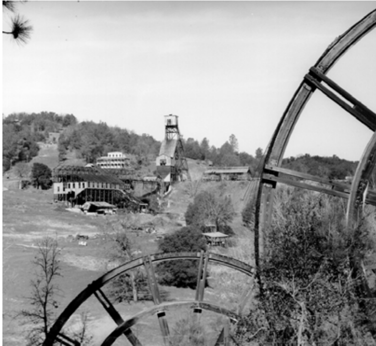
Figure 9: Tailings Wheels at Kennedy Mine, Amador County, n.d. Tailings wheels (68 ft. tall) used to transport wastes for storage (used with permission, California Department of Conservation, California Geological Survey).
