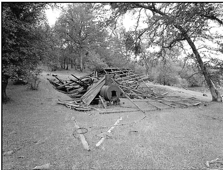
Figure 51: Tractor-boiler that Supplied Power to Two-stamp Mill at Defiance Claim (Library of Congress, HAER Photo by Alice Olmstead).
