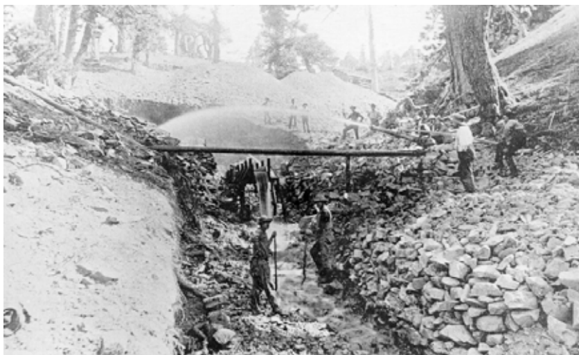
Figure 22: Low-level Hydraulic Mining at the Hocumac Mine, San Bernardino County 1895 (used with permission, California Department of Conservation, California Geological Survey).
