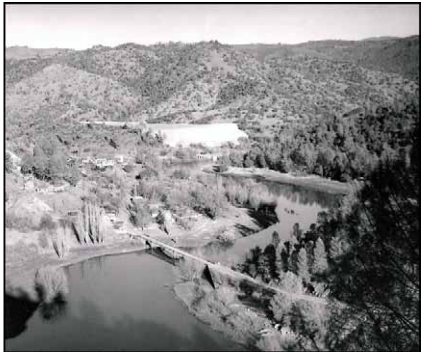
Figure 59: Tailings at New Melones Reservoir, Stanislaus River Drainage. The mill tailings were slurried to a neighboring valley resulting in the white fill visible in background. (Courtesy Calaveras County Historical Society).
