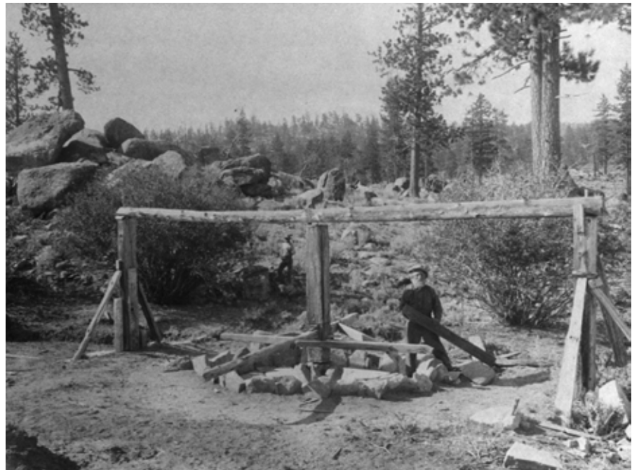
Figure 29: Arrastra in the High Sierra, circa 1900 (used with permission, California State Department of Conservation, California Geological Survey).
