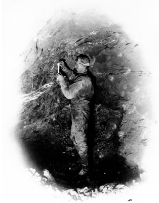
Figure 39: Blasting at Empire Mine, Nevada County, 1900. Miner is splitting (lighting) a fuse with a candle 2100-ft. underground (used with permission, California Department of Conservation, California Geological Survey).
