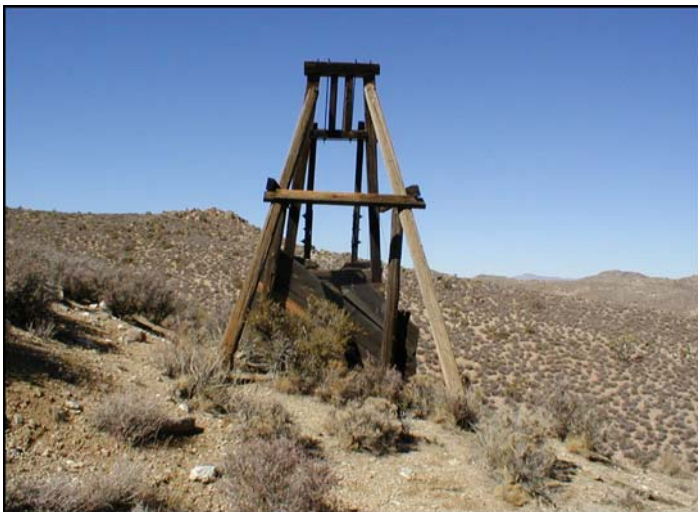
Figure 53: Small Head Frame with Chute, Inyo County (Courtesy JRP Historical Consulting Services).
