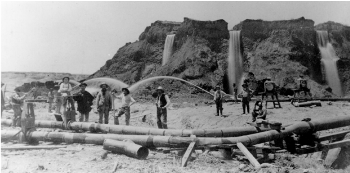
Figure 24: Hydraulic Mining at Michigan Bar, Sacramento County 1860. Waterfalls in background are ground sluices. Locomotive lamps to right of frame are for nighttime flood lights (used with permission, California Department of Conservation, California Geological Survey).
