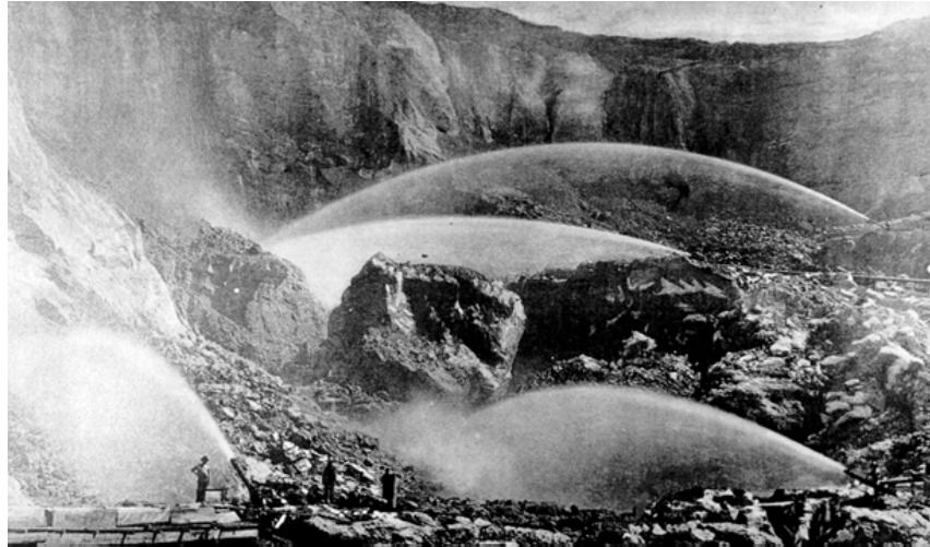
Figure 25: North Bloomfield Mine (Malakoff Diggings), Nevada County, 1890 (used with permission, California Department of Conservation, California Geological Survey).
