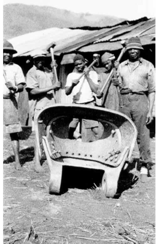
Figure 35: Andrada Dredge Mine, African-American crew with new lip applied to clam shell bucket, circa 1930s (used with permission, California Department of Conservation, California Geological Survey).
