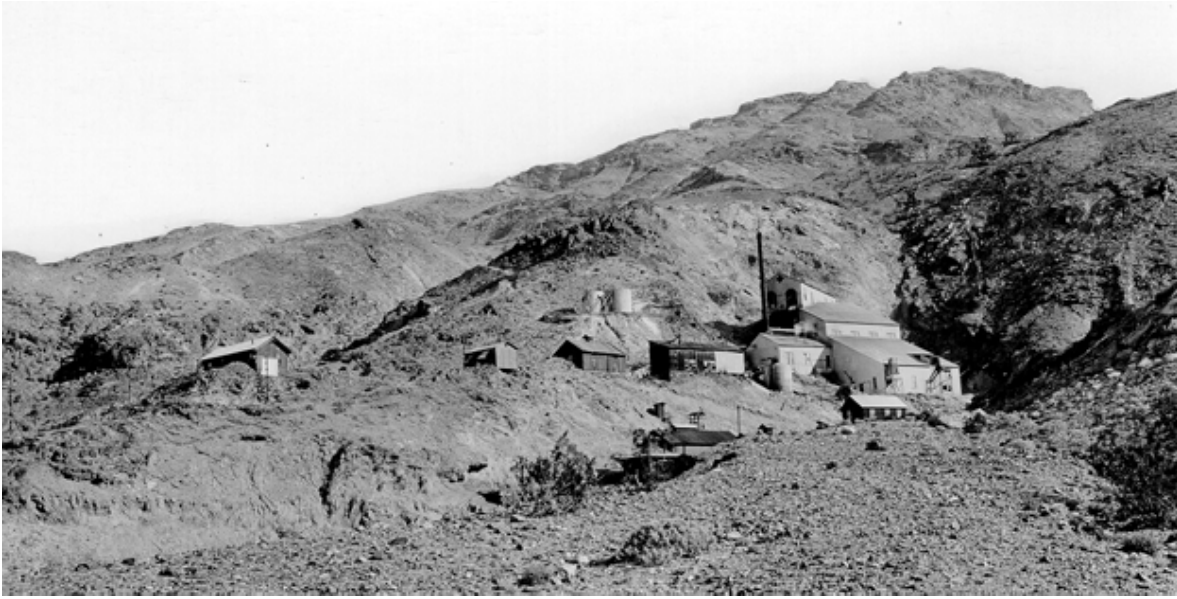
Figure 10: Keane Wonder Mine, Inyo County, 1916. Said to have produced $1,100,000 before closing in 1916 when ore was depleted (used with permission, California Department of Conservation, California Geological Survey).
