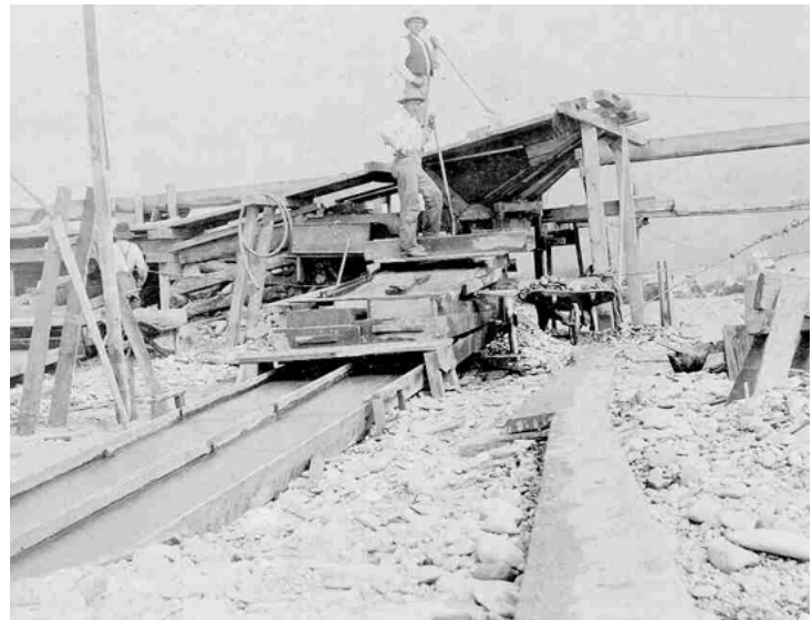
Figure 8: Lower Gold Bluff Mine, Humboldt County, 1895. Oregon tom (long tom) saving gold on bare boards (used with permission, California Department of Conservation, California Geological Survey).
