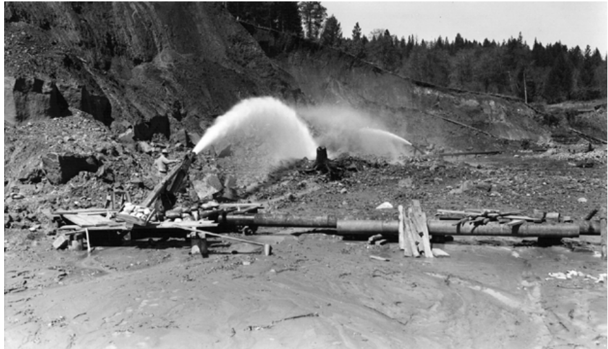
Figure 6: Hydraulic Mining, Junction City, Trinity County, n.d. (used with permission, California Department of Conservation, California Geological Survey).
