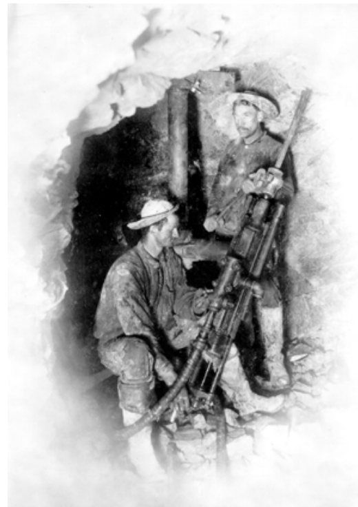
Figure 40: Air Drill Operators, Empire Mine, Nevada County, ca. 1900. Two miners drifting (that is, following the vein) with an air-driven machine drill 2100-ft. underground (used with permission, California Department of Conservation, California Geological Survey).
