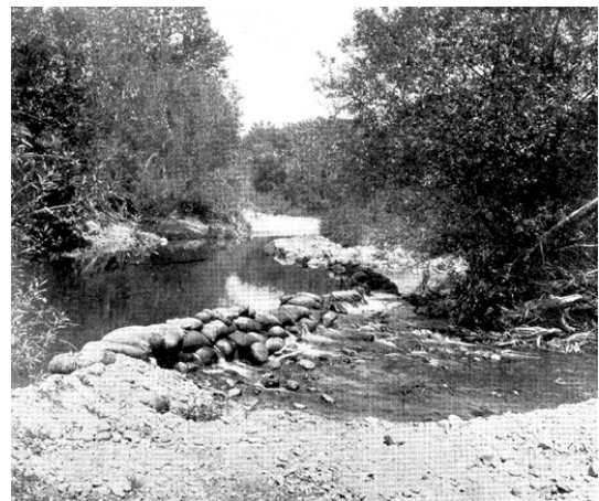
Figure B1. Temporary cobble diverting weir, Vandalia Ditch, circa 1900 (Mead 1902, Bulletin No. 119:Plate 26)
