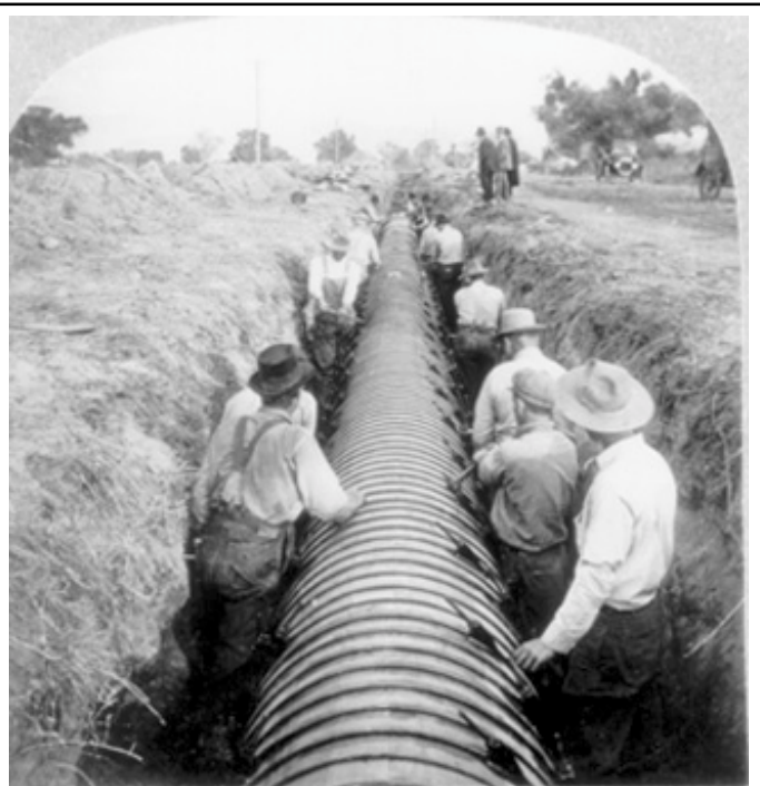
Figure B10. Wood stave pipe construction (California Room, California State Library)
