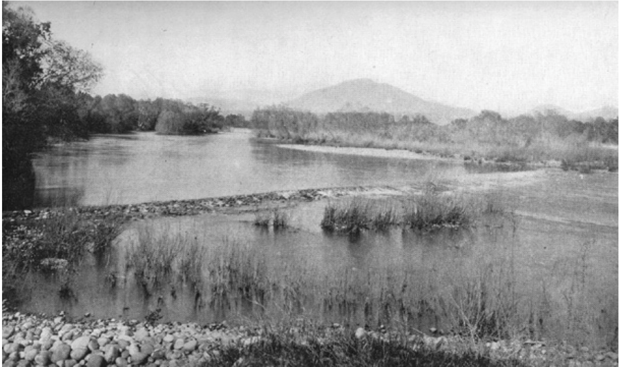
Figure 5. Cobble and brush dam, Fresno Canal, ca. 1898 (Grunsky 1898, Water Supply Paper No. 18:46)
