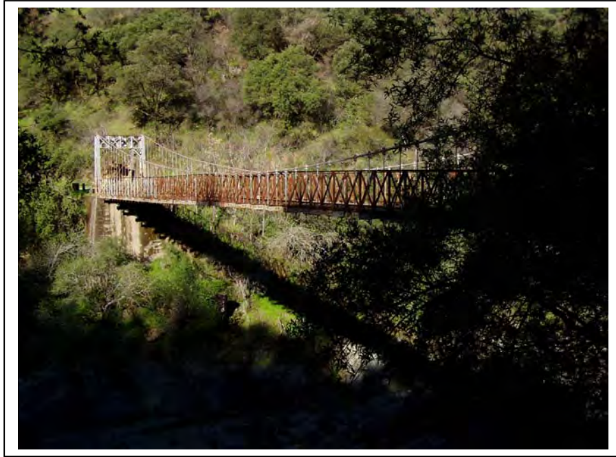
Bridge 19C0002, Colfax-Forrest Hill Road, North Fork American River, March 2003
