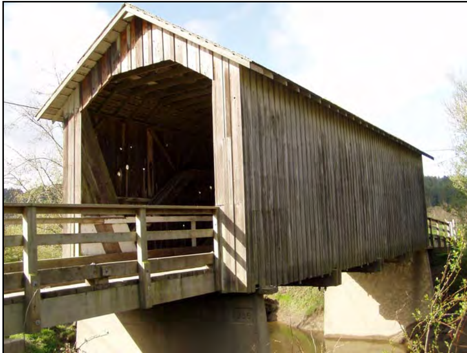
Photograph 4: Berta’s Ranch Road Bridge (04C0047). Howe truss covered bridge built in 1936.
