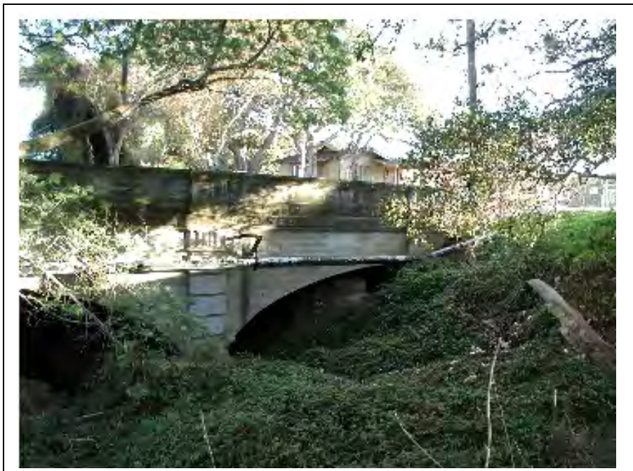
Bridge 44C0082, Larkin Street, Hartnell Gulch, June 2003
