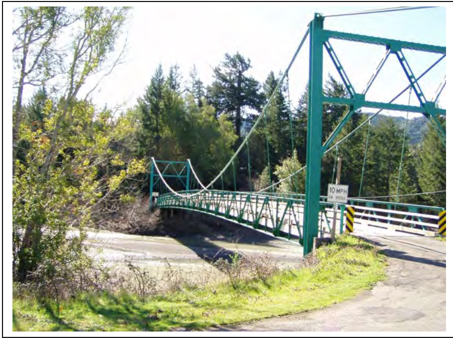
Bridge 04C0075, Lindley Road, Mattole River, February 2003
