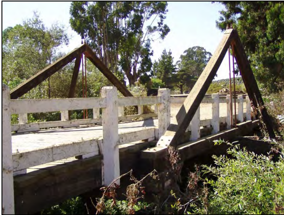
Photograph 2: Cayucos Creek Bridge (49C0248). A-Frame truss built in 1940.
