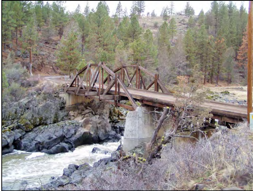
Photograph 5: Stone Coal Bridge (3C0092). Camelback truss built in 1953.
