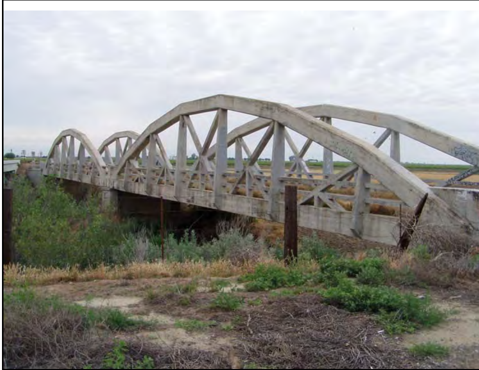
Photograph 9: Murphy Slough Bridge (42C0551Z), constructed in 1916.
