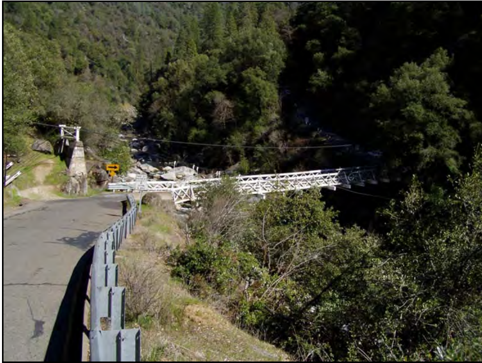
Photograph 6: Mosquito Bridge (25C0061). Timber suspension bridge built in 1939.
