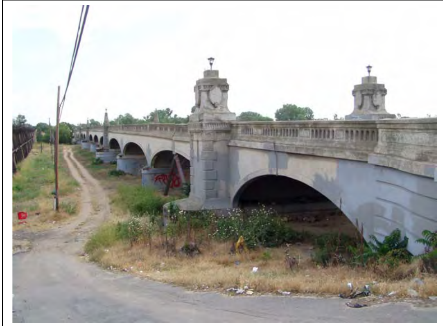
Bridge 38C0023, Seventh Street, Tuolumne River, May 2003
