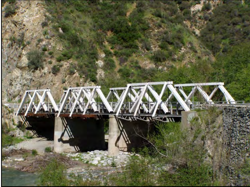
Photograph 1: Cattle Canyon Creek Bridge (53C0972)
