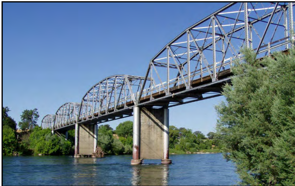
Photograph 7: Jellys Ferry Road Bridge (08C0043) over Sacramento River, built 1949. Example of a Parker truss. June 2003.
