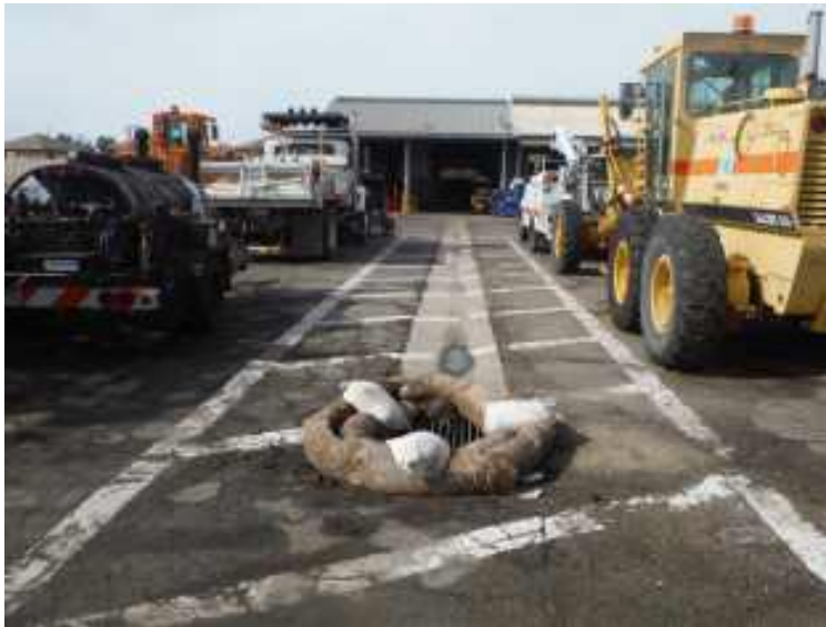
Figure C.5-1 Storm Drain Inlet Protection
