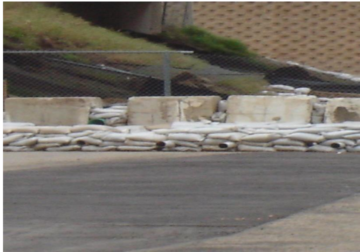
Figure C.4.2-1 Gravel bag Barrier
