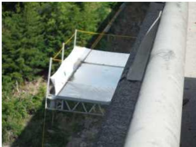
Bridge work area over water lined with plastic sheeting
