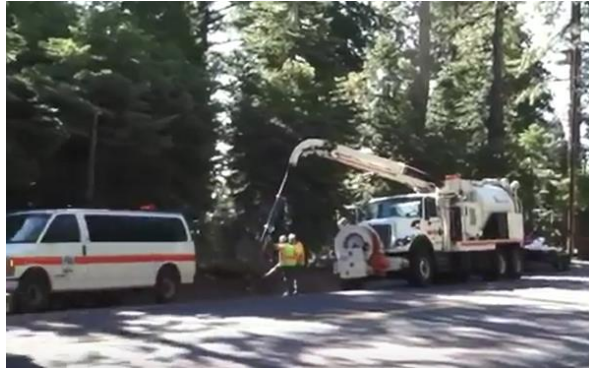
Figure C.22.1-1 Baseline Stormwater Drainage Facilities Inspection and Cleaning
