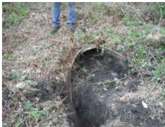
Culvert scheduled for cleaning
