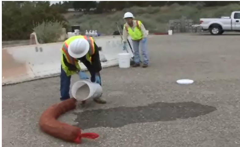
Figure C.13.1-1 Spill Prevention and Control
