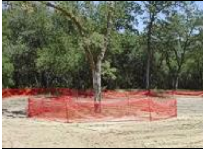
Figure C.8-1 Preservation of Vegetation
