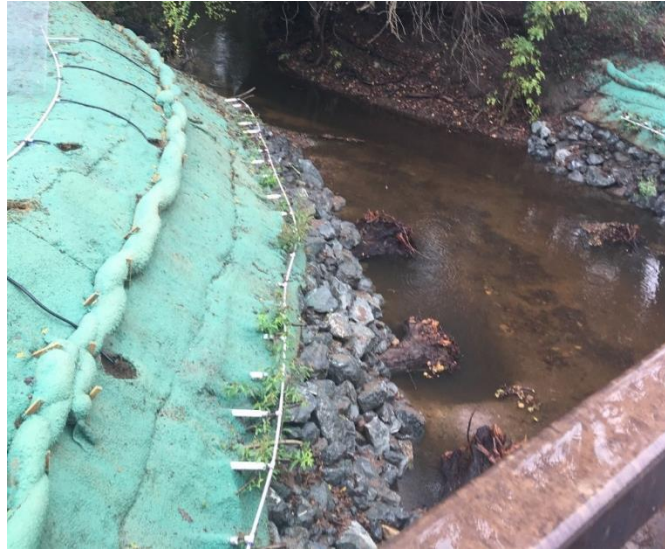
Figure C.4.4-1 Fiber Rolls used to break slope length
