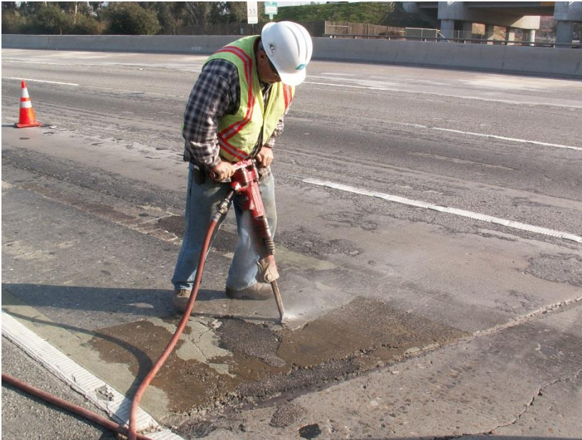
Concrete slab repair
