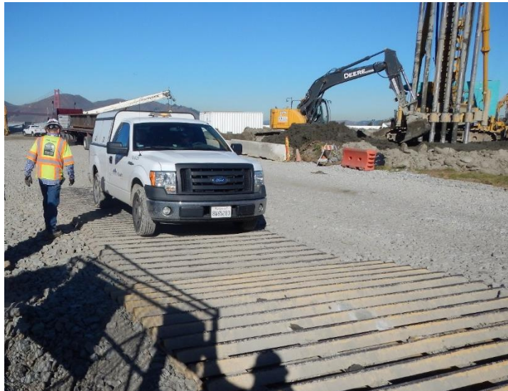
Figure C.12-1 Stabilized Activity Entrance/Exit
