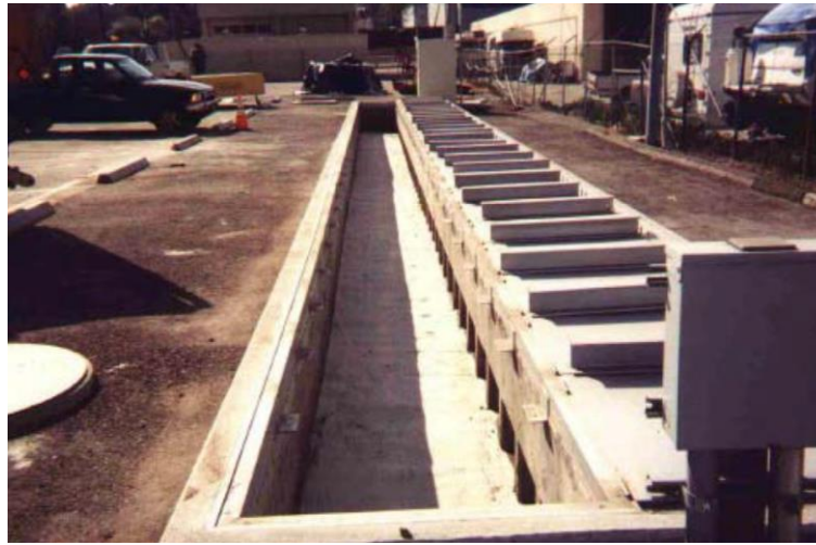
Figure C.23.8-1 Delaware Sand Filters
