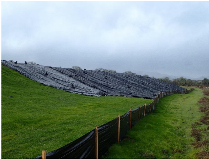
Figure C-4.1. Silt Fence for Stockpile Perimeter Control
