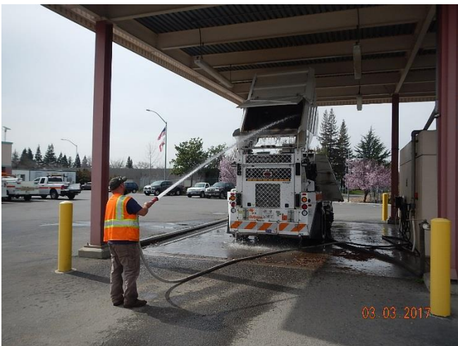
Washwater contained in wash rack
