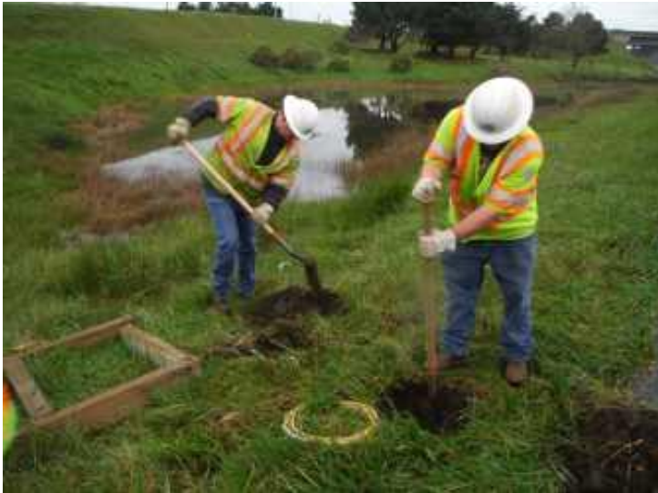
Post holing for new sign
