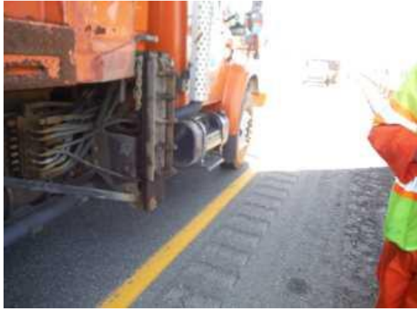
Sealing operation; no leaks/drips observed
