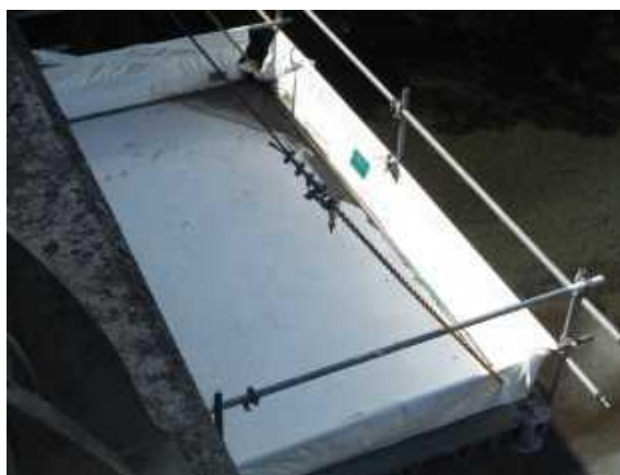
Work area over water; plastic sheet containment
