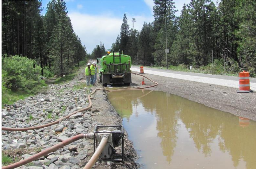
Figure C.28-1 Dewatering Operation
