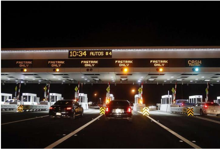
Clean toll booth lanes
