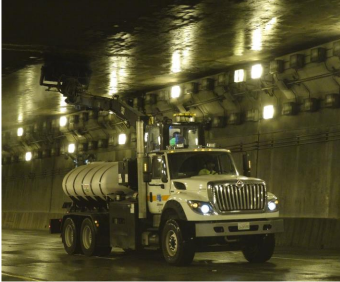
Washing tunnel wall
