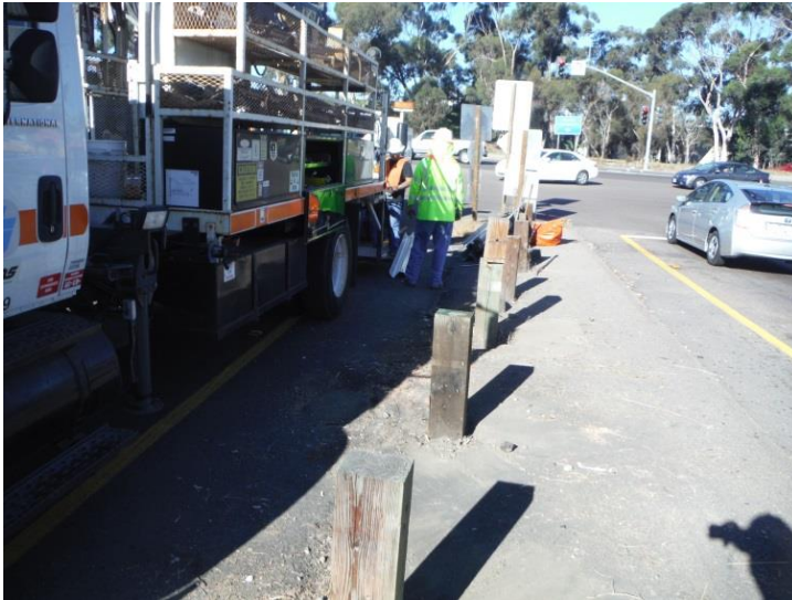
Guardrail repair in progress
