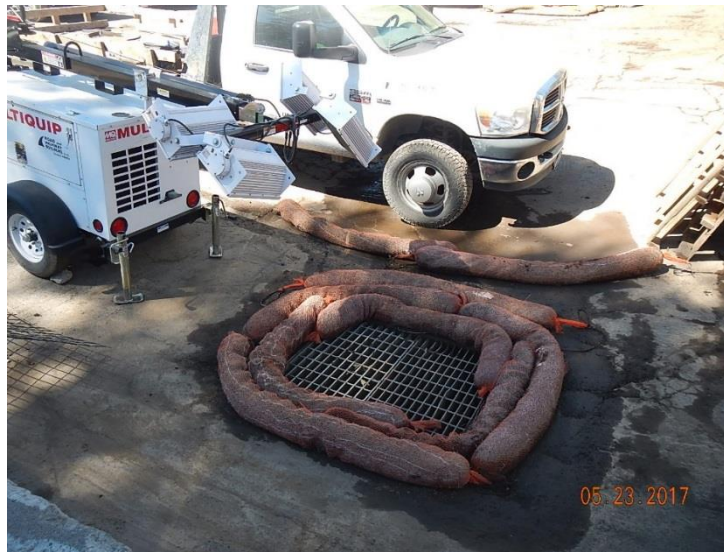
Figure C.4.7-1 Fiber Rolls Used as Check Dams and for Drain Inlet Protection
