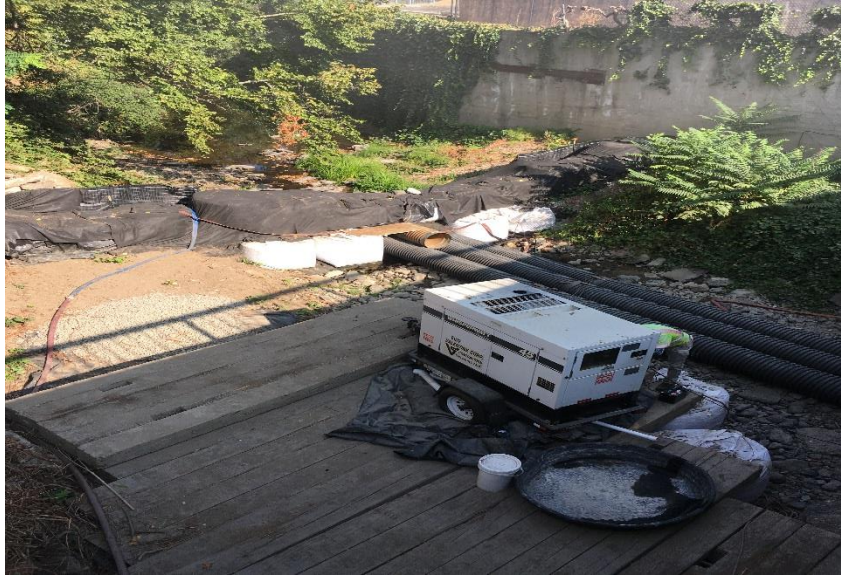
Figure C.10-1 Work in a Waterbody
