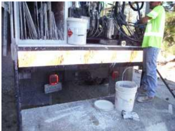
Epoxy pavement markings operation
