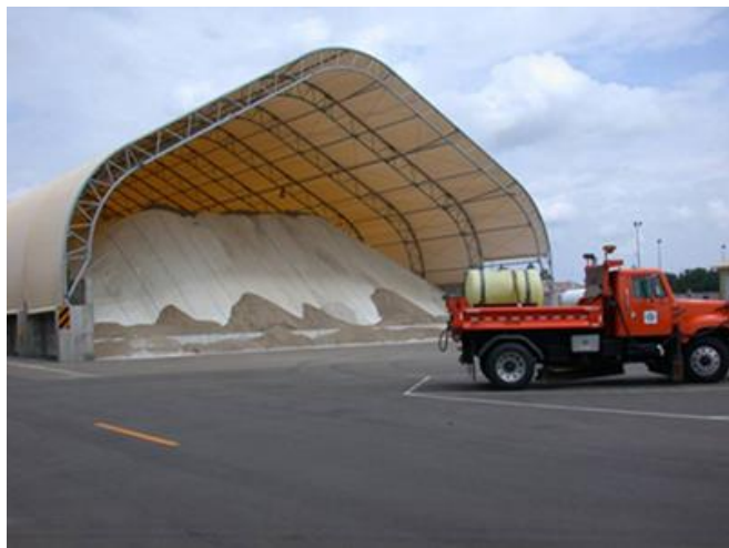
Salt storage house
