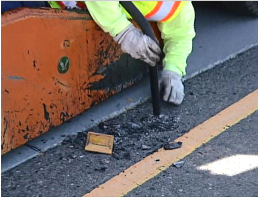
Removing recess marker
