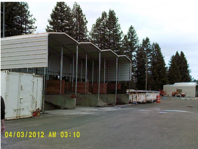
Materials stored in covered sheds, bins or shipping containers
