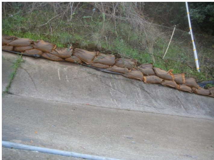
Gravel bag berm protection at concrete-lined channel
