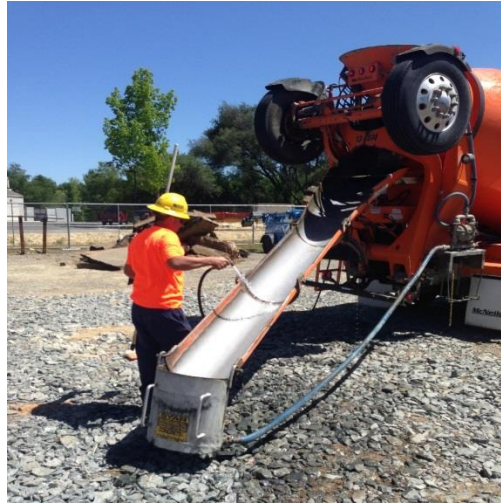
Figure 13.7-1 Concrete Waste Management
