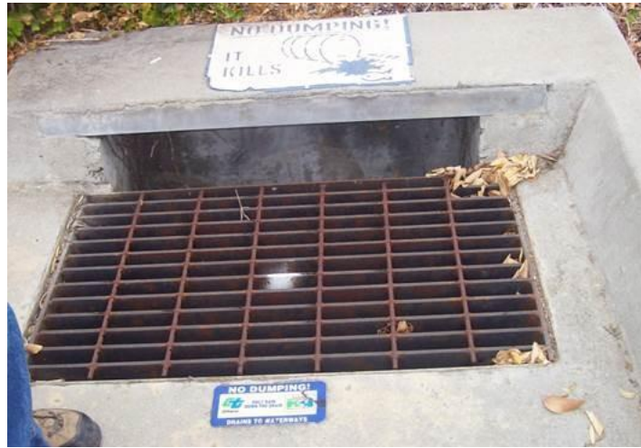
Figure C.20.1. Stenciled Storm Drain
