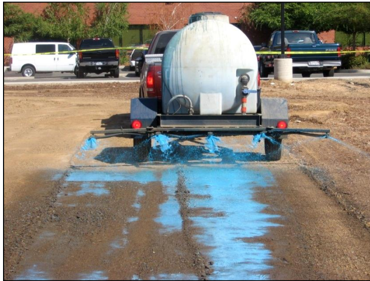
Figure C.7.5-1 Soil Binder Application
