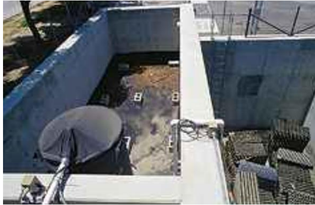
Figure C.23.9-1 Multi-Chambered Treatment Train
