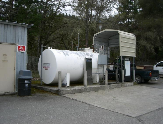
Fueling station well maintained; no concrete staining
