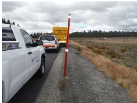
Snow pole installation
