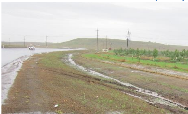
Shoulder graded; slope with netting and hydroseeding
