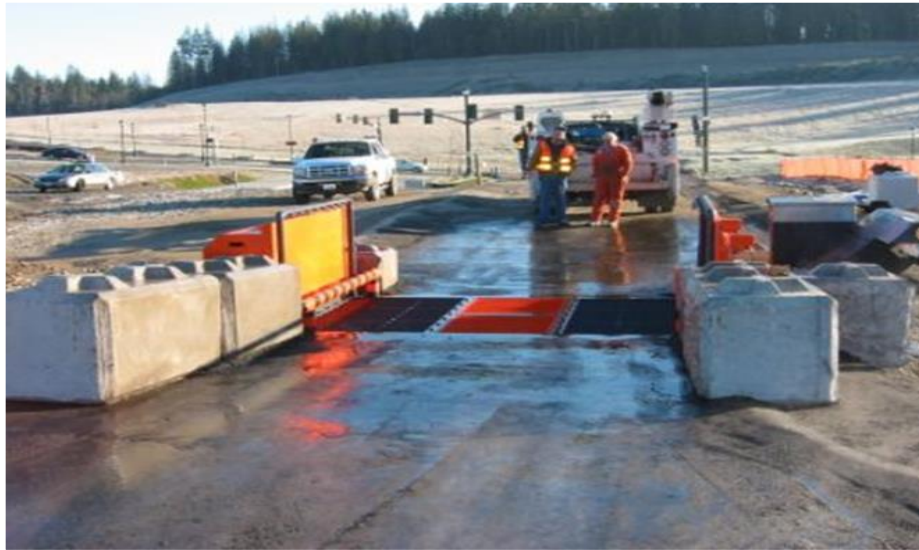
Figure C.12.2-1 Tire Inspection and Sediment Removal
