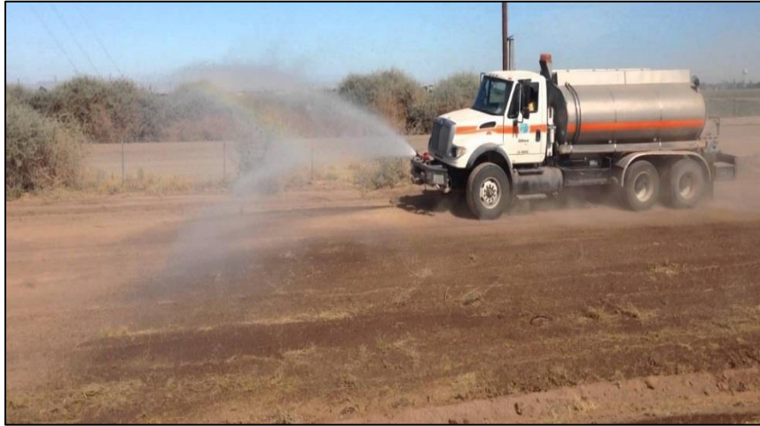
Figure C.11-1 Wind Erosion Control
