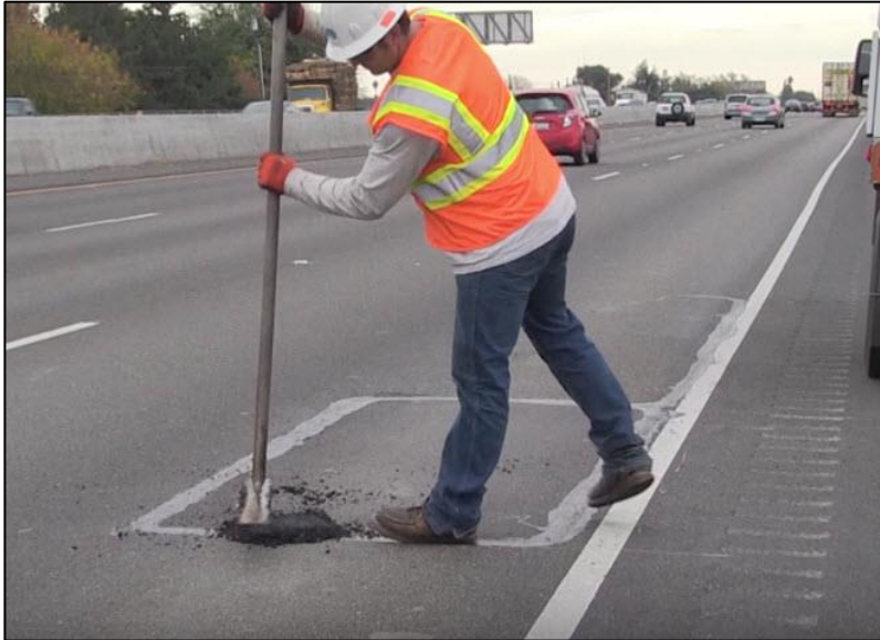
Pothole repair
