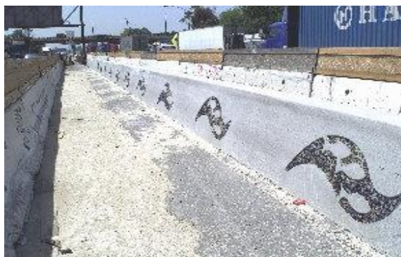
Sandblasting to etch median barrier
