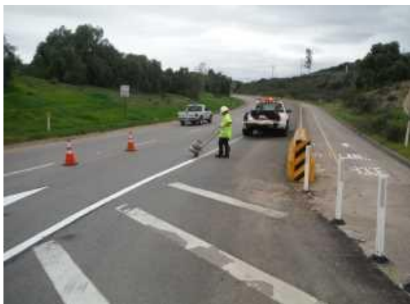
Applying thermoplastic strips with a propane heater
