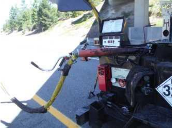
Sealing operation; no leaks observed
