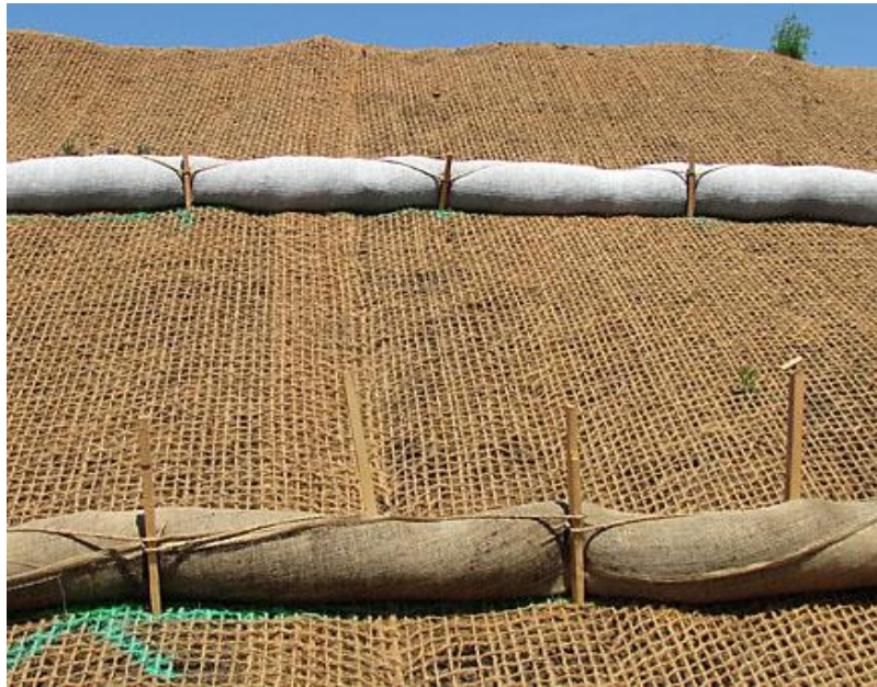
Figure C.4.8-1 Compost sock with jute netting
