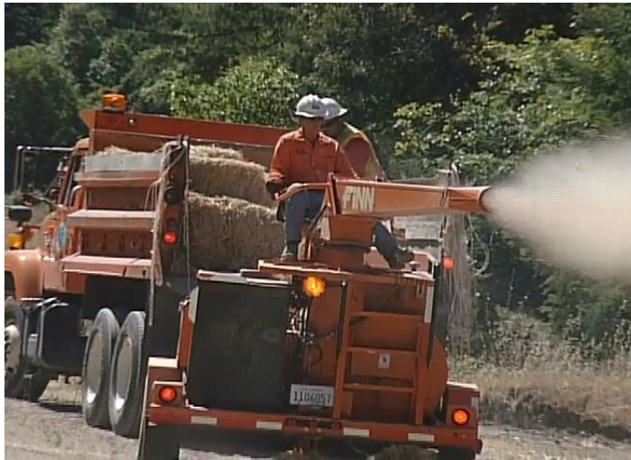
Figure C.7.6-1 Straw Mulch Application
