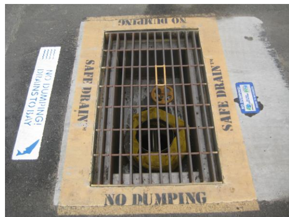
Facility storm drain stenciling downgradient of hazardous waste storage lockers
