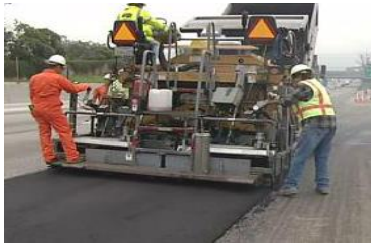
Figure C.16. Paving operations procedures
