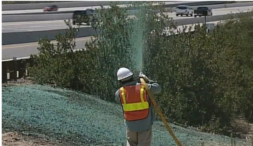
Figure C.7.4.-1 Hydroseeding Application
