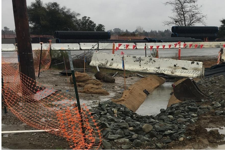
Figure C.6.3.-1 Temporary Diversion Ditches
