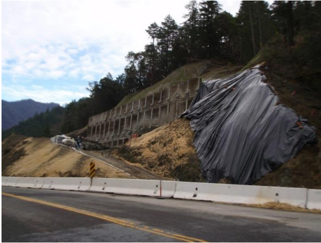
Slide area swept and temporarily repaired with plastic sheeting
