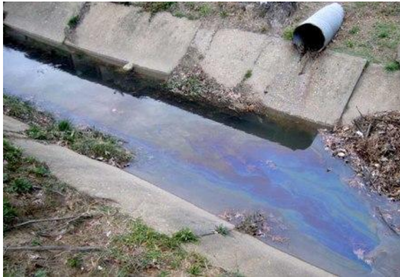
Figure C.22.4-1 Illegal Spill Discharge
