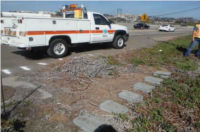
Work area clean and well maintained
