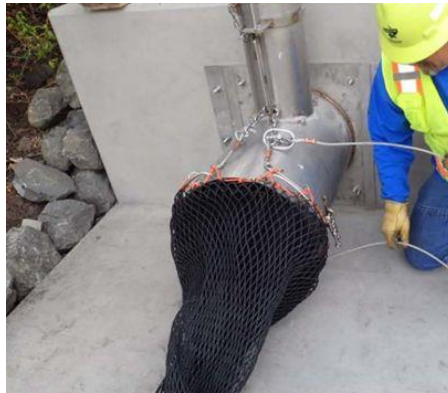
Figure 15-1 Attaching the Bag Retention Cable
