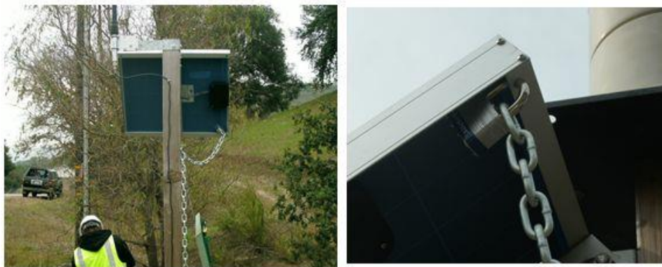
Figure 8-11 Secure Solar Panel Installation
