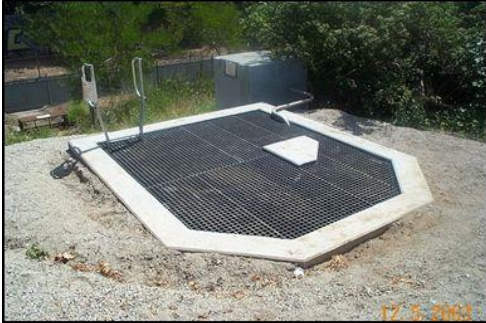
Figure 15-4 Example of Inclined Screen GSRD
