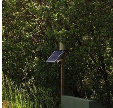
Figure 8-9 Rain Gauge Blocked by Foliage
