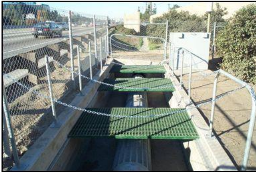
Figure 15-6 Example of Linear Radial GSRD, View #1
