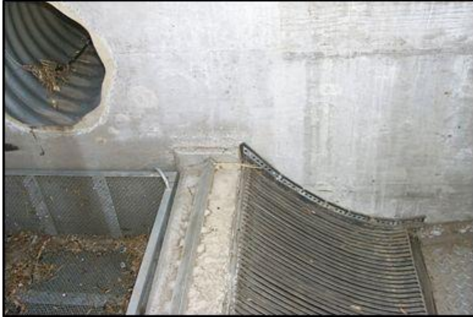
Figure 15-8 Example of Parabolic Screen GSRD
