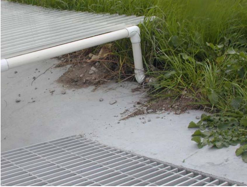
Figure 7. Gopher Activity at Edge of Collection Ditch at Irvine
