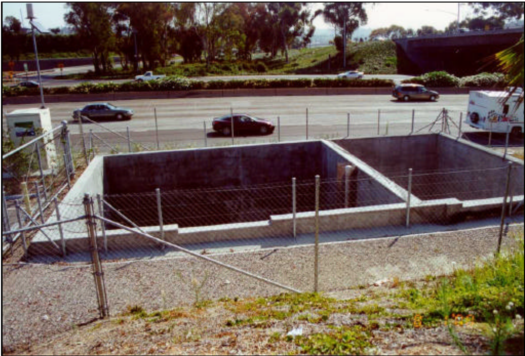
Figure 2-2 I-5/SR-78 Austin Sand Filter
