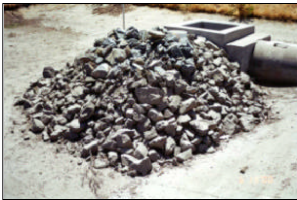
Figure 3-2 District 7 Outlet Riser
