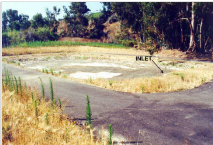
Figure 5-1 I-5/La Costa Infiltration Basin
