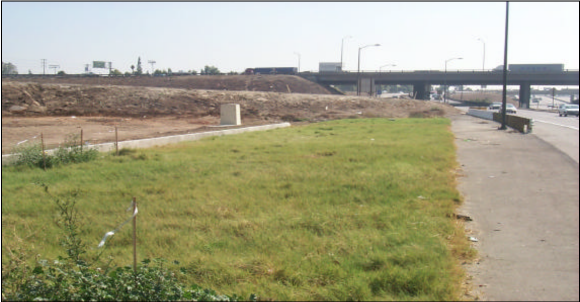
Figure 8-1 Biofiltration Strip (District 7, I-605/SR-91)
