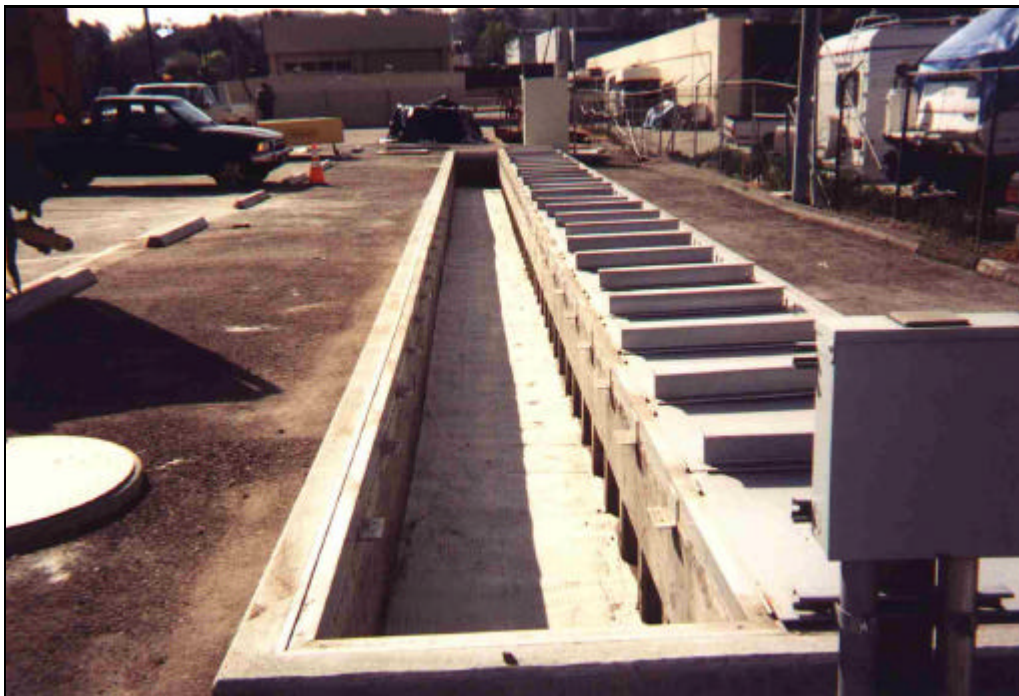
Figure 2-4 Escondido MS Delaware Sand Filter
