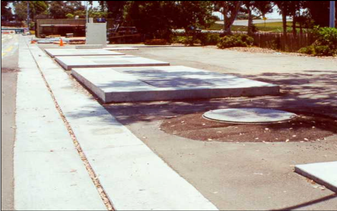
Figure 9-2 Surface View at Kearny Mesa
