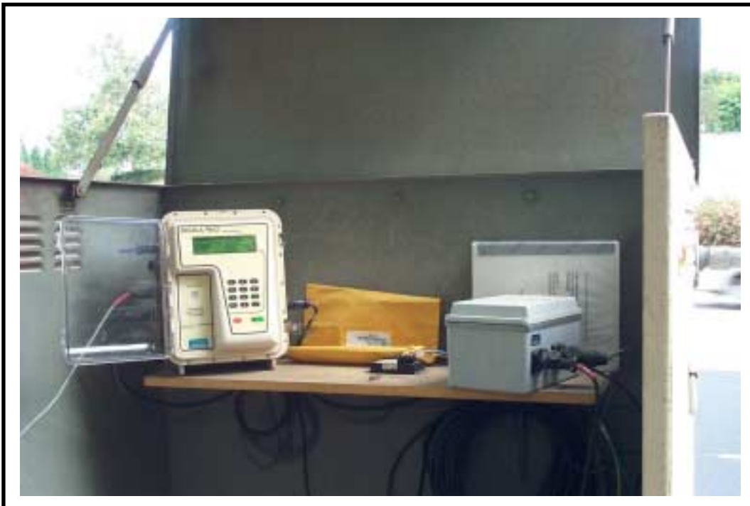
Photo No. 3 – Sigma Flowmeter, Mobile Phone and Encroachment Permit at Site 01
