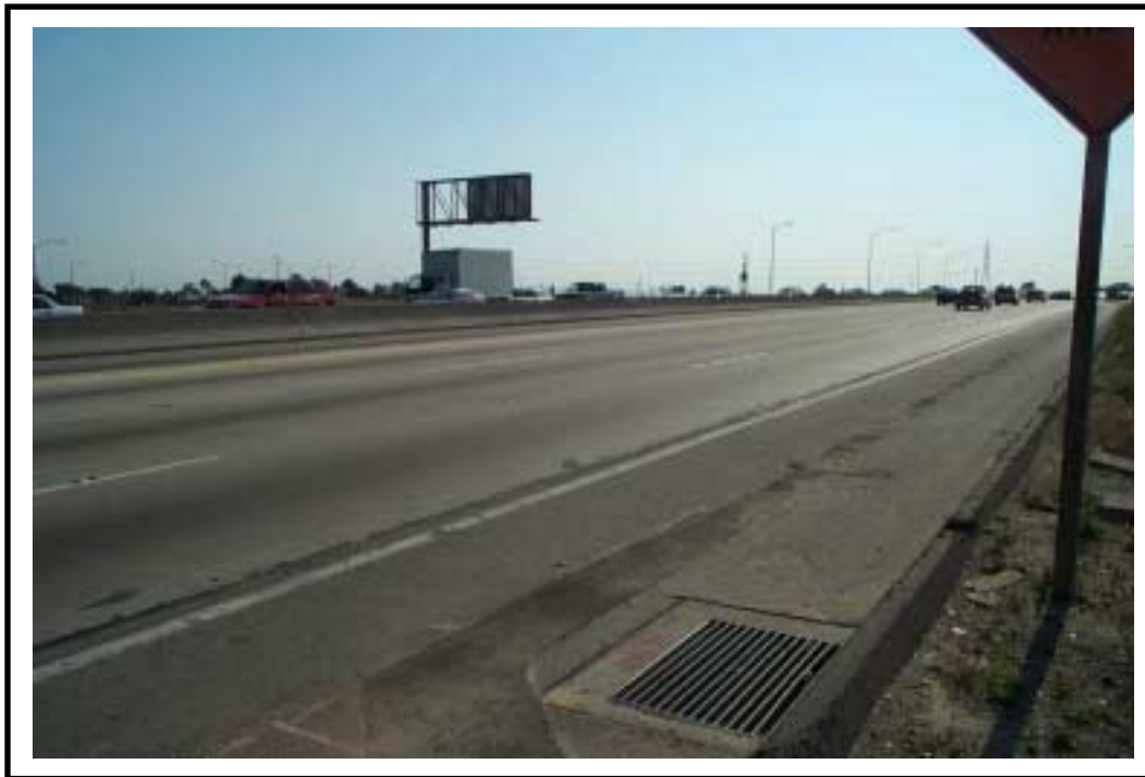
Photo No. 2 – Section of W/B 91 Freeway at Site 14
