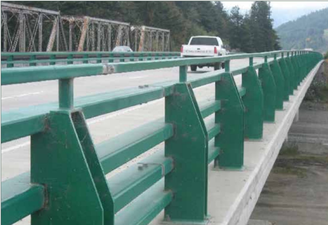
Exterior view of above.
