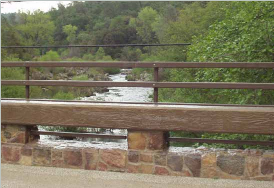
Photo of Concrete Barrier Type 80 modified with architectural treatment and 54-inch-high bicycle rail offset 15 inches from barrier rail face on the Bear River Bridge on the Placer/Nevada County line. (03-PLA-049-PM 011.35)
