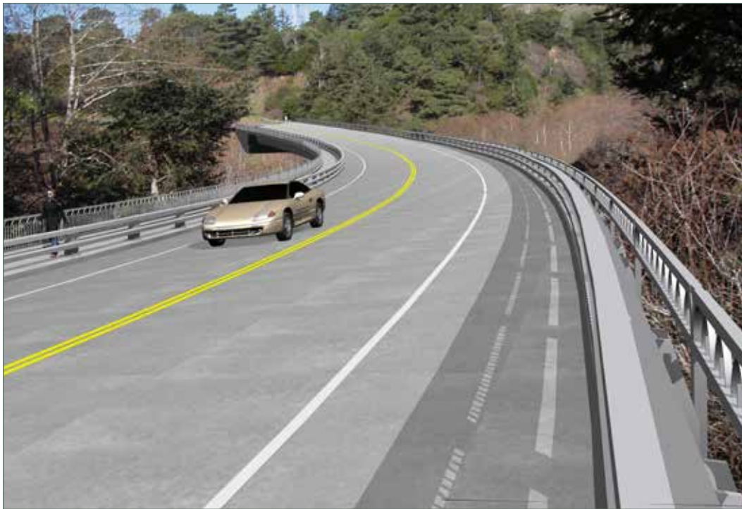
Rendering of 42-inch-high California ST-10 Bicycle Rail on the right and ST-10 / pedestrian walkway / 42-inch-high pedestrian rail on the left at Greenwood Creek Bridge in Mendocino County. (01-MEN-001-PM 033.7)
