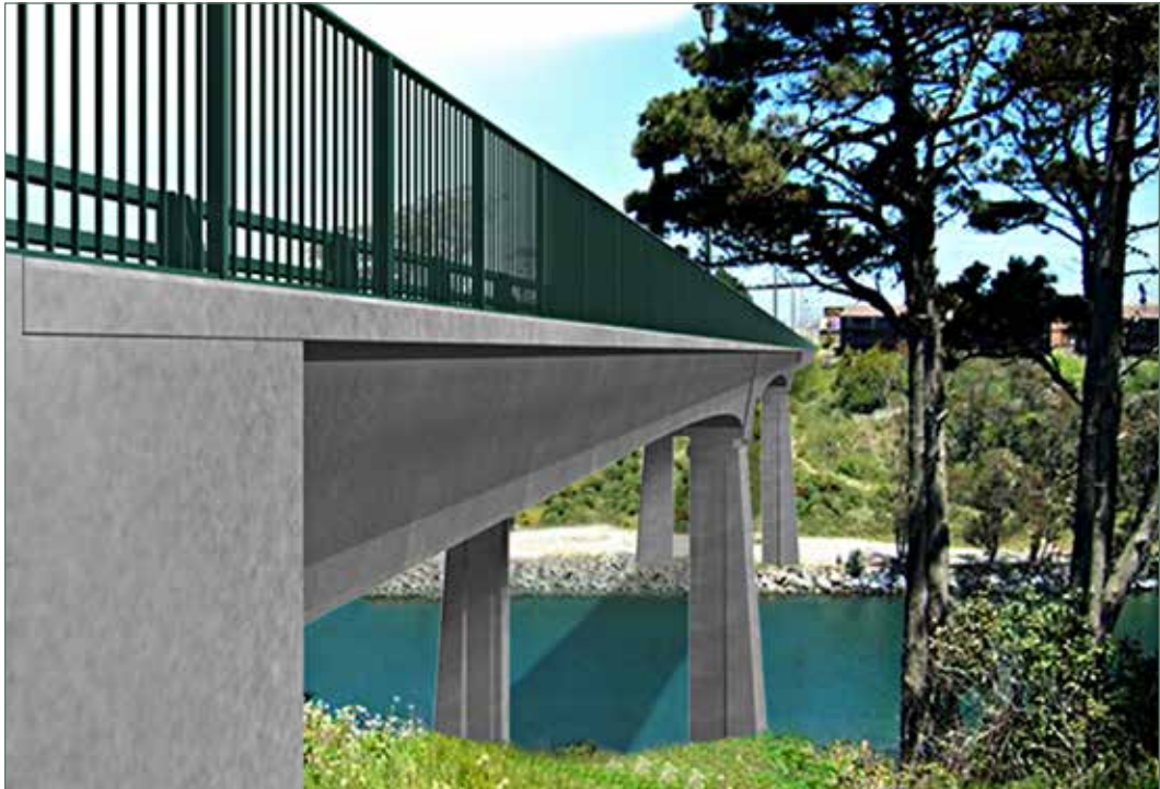
Rendering of California ST-10 Bridge Rail with sidewalk and steel pedestrian handrail at Noyo River Bridge on State Route 1 at Fort Bragg in Mendocino County. (01-MEN-001-PM 060.2)
