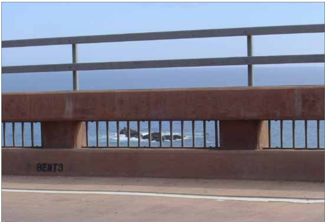
Photo of Concrete Barrier Type 80 modified with color, 54-inch-high bicycle rail, and lower clear opening size reduced for bicycle traffic on the Forest Boundary Viaduct in Monterey County. (05-MON-001-PM 001.49)
