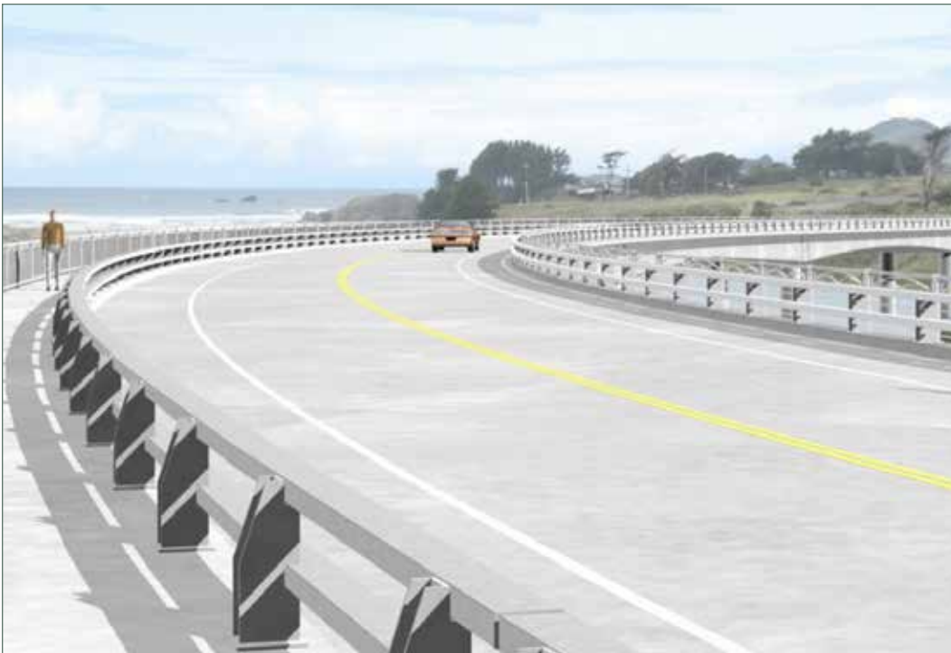
Rendering of Ten Mile River Bridge in Mendocino County with California ST-10 Bridge Rail with a pedestrian walkway and 42-inch-high handrail on the coastal side of bridge and 42-inch-high bicycle rail on the inland side. (01-MEN-001-PM 069.7)
