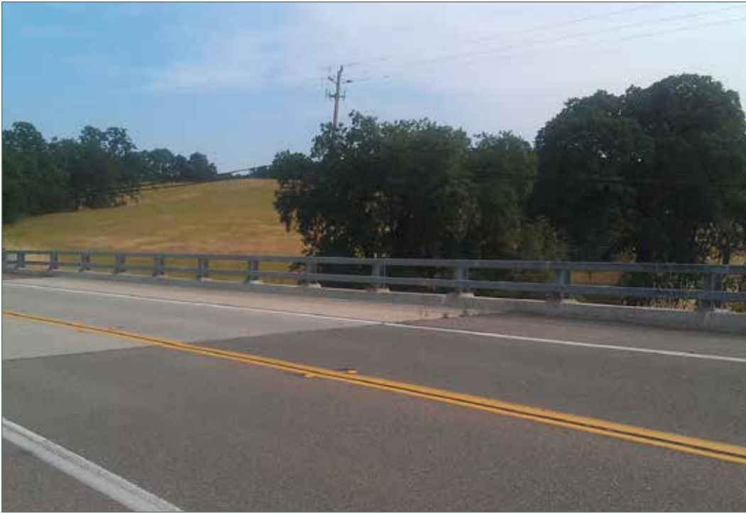
Photo of interior view of California ST-30 Bridge Rail at the South Fork Dibble Creek Bridge in Tehama County. (02-TEH-036-PM 39.0)
