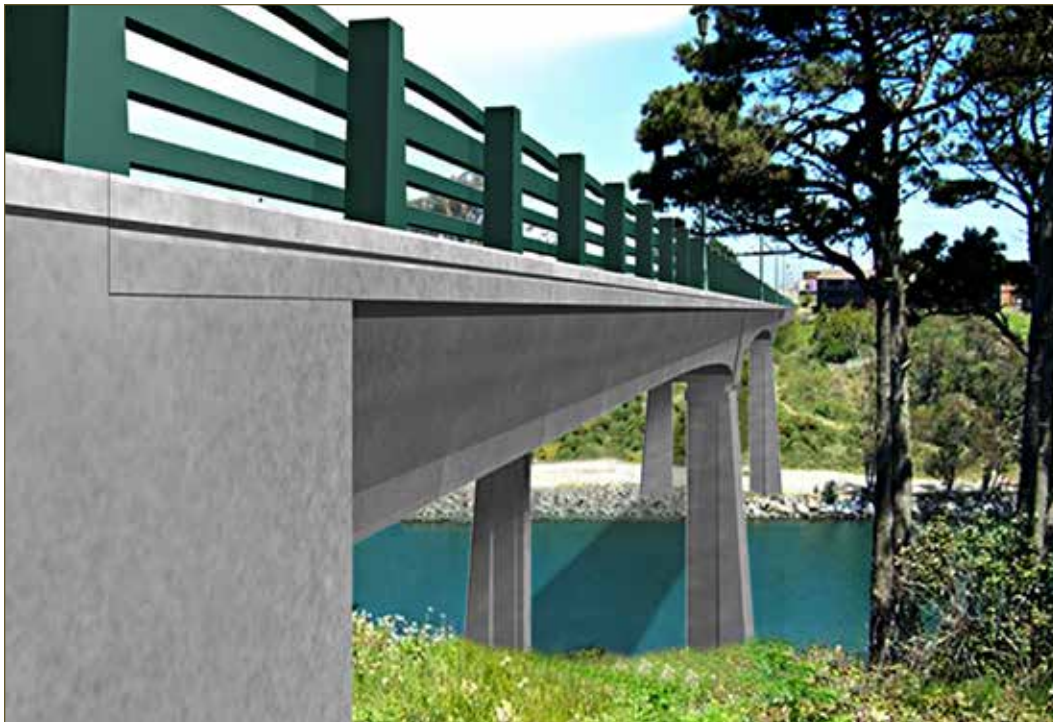
Rendering of California ST-40 Bridge Rail modified with arched top bar and vertical posts that flare from top to bottom. This is one of the bridge rail alternatives that was considered for the Noyo River Bridge in Mendocino County. (01-MEN-001-PM 060.2)
