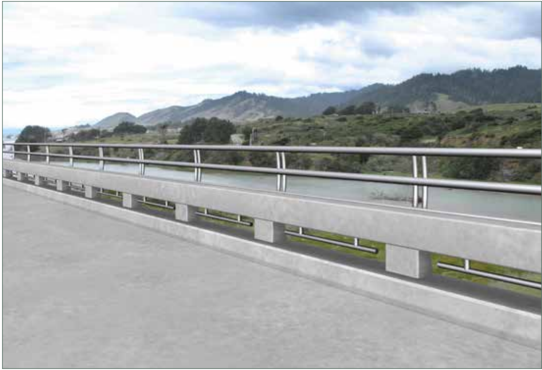
Rendering of Concrete Barrier Type 80 in an unspecified location with an alternative 54-inch-high bicycle rail and alternative design for reducing lower clear opening in concrete to conform to bicycle requirements.
