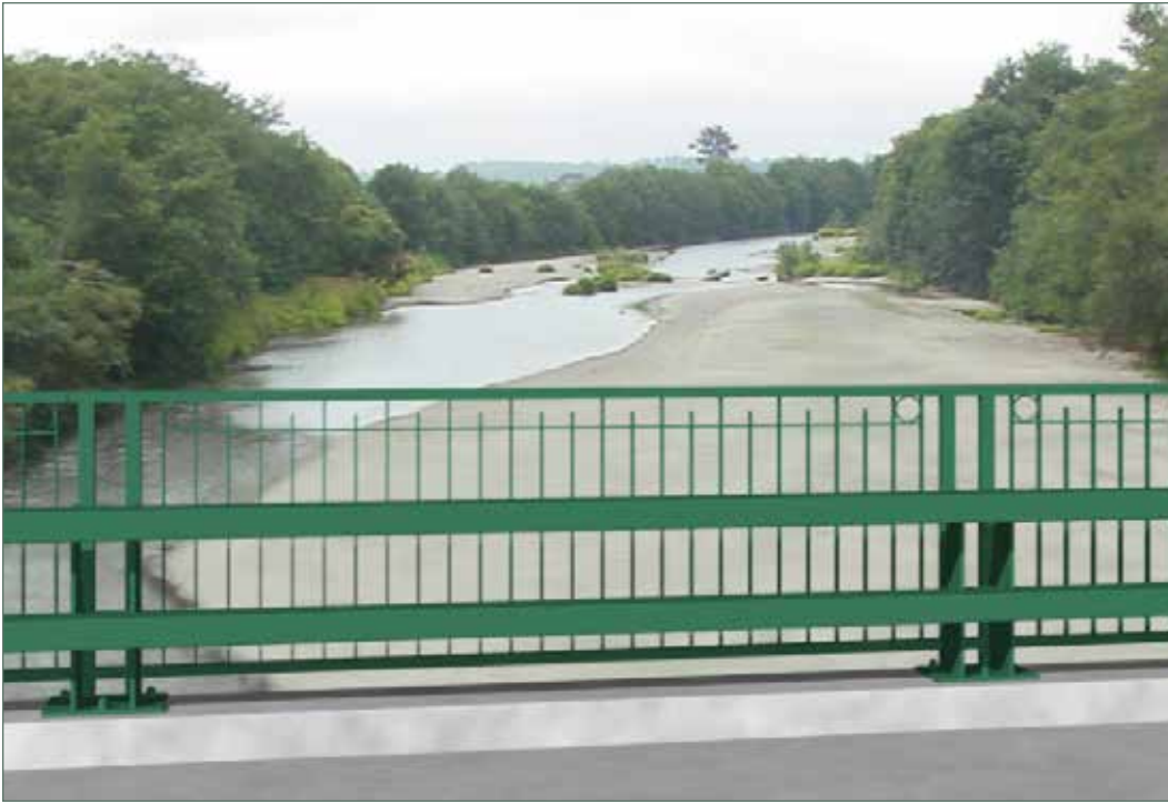
Rendering of 42-inch-high California ST-10 Bicycle Rail on Mad River Bridge in Humboldt County. (01-HUM-101-PM 090.8)
