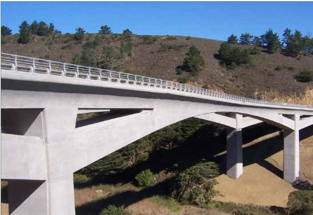
Exterior view of Concrete Barrier Type 80 with custom 54-inch-high bicycle rail on the Devil's Slide Bridges on the north end of the Devil's Slide Tunnel. (04-SM-001-PM 39.66)
