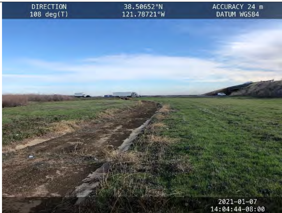
Photo 6. View to east of Feature 03, a canal.
