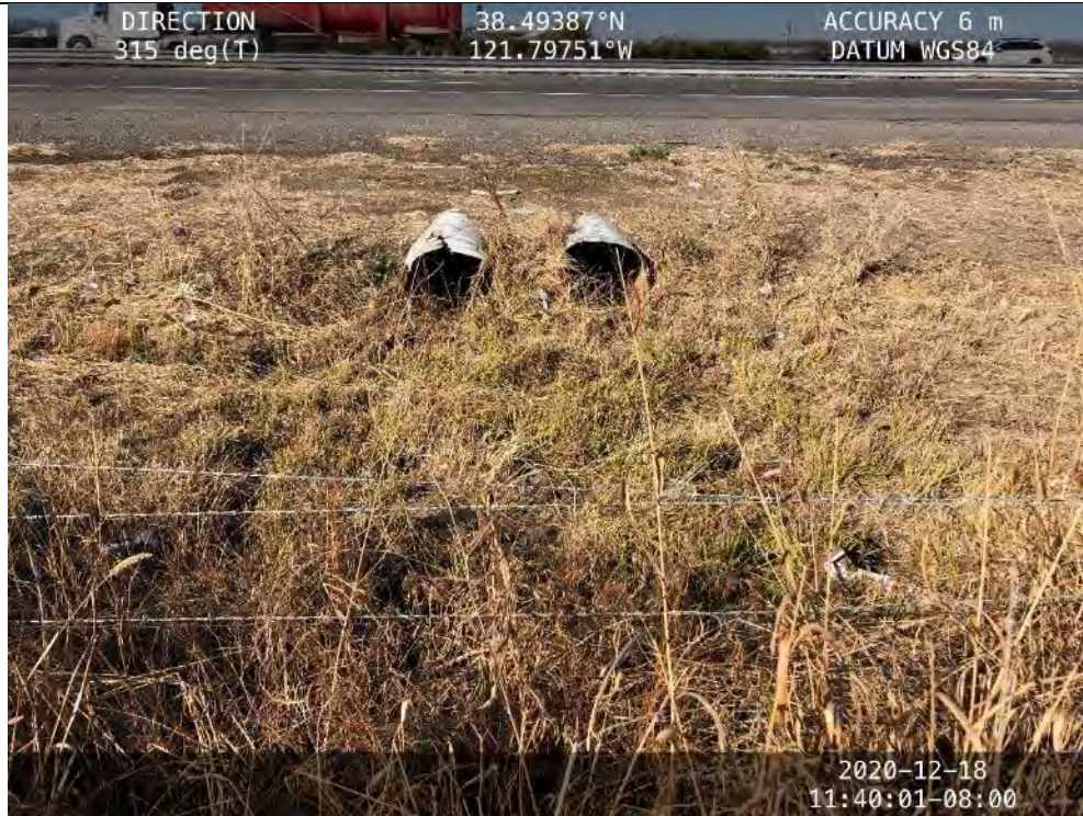
Photo 3. View to the northwest of roadside culvert.
