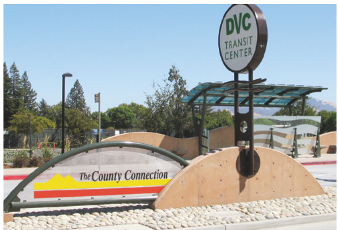
A new transit center at Diablo Valley College in Pleasant Hill (Contra Costa County) was built through Prop. 1B, one of the many smaller projects throughout the state that received bond funding.
