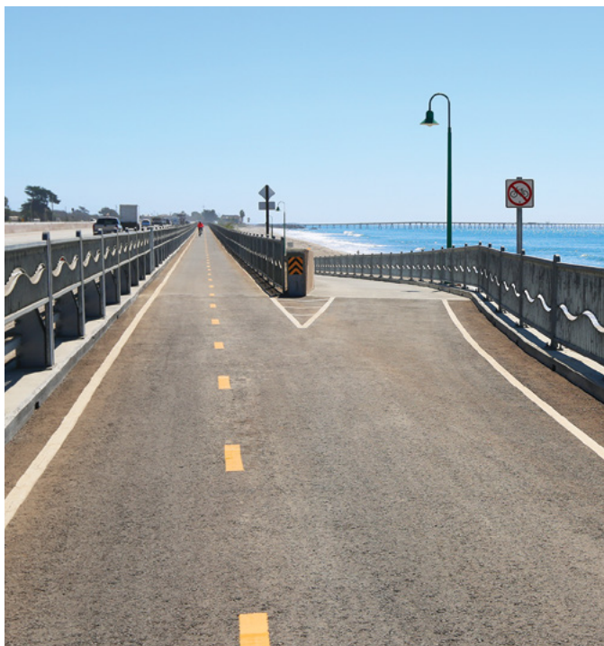
The bike path and pedestrian undercrossing at La Conchita, along U.S. Highway 101 in Ventura County, were completed in 2014.
