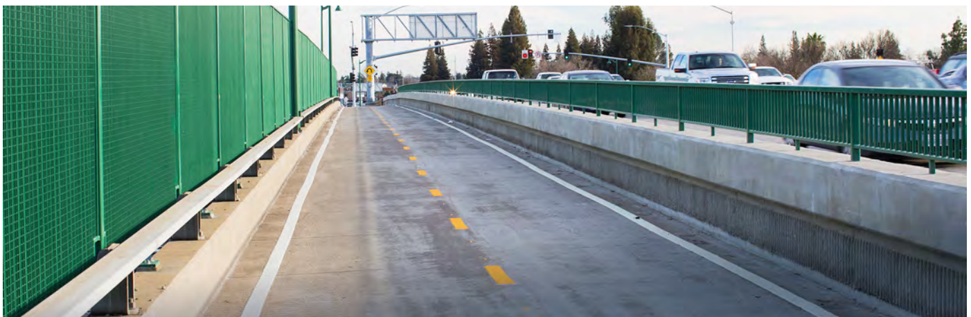
A concrete-and-steel barrier separates vehicular traffic from cyclists on this Class 1 bicycle path over Highway 50 in Sacramento. The bicycle and pedestrian projects funded by the Active Transportation Program not only encourage increased use of active modes, they support sustainable communities and healthier, low-carbon travel choices.
