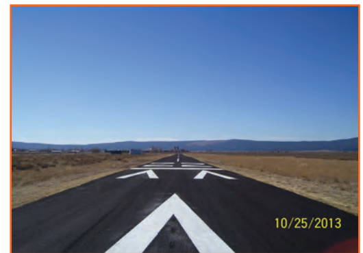
Runway After Construction
