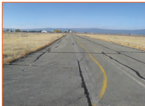
Runway Before Construction
