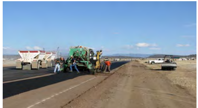
During: Pavement Overlay Construction
