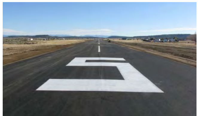
After: Newly Paved and Marked Runway
