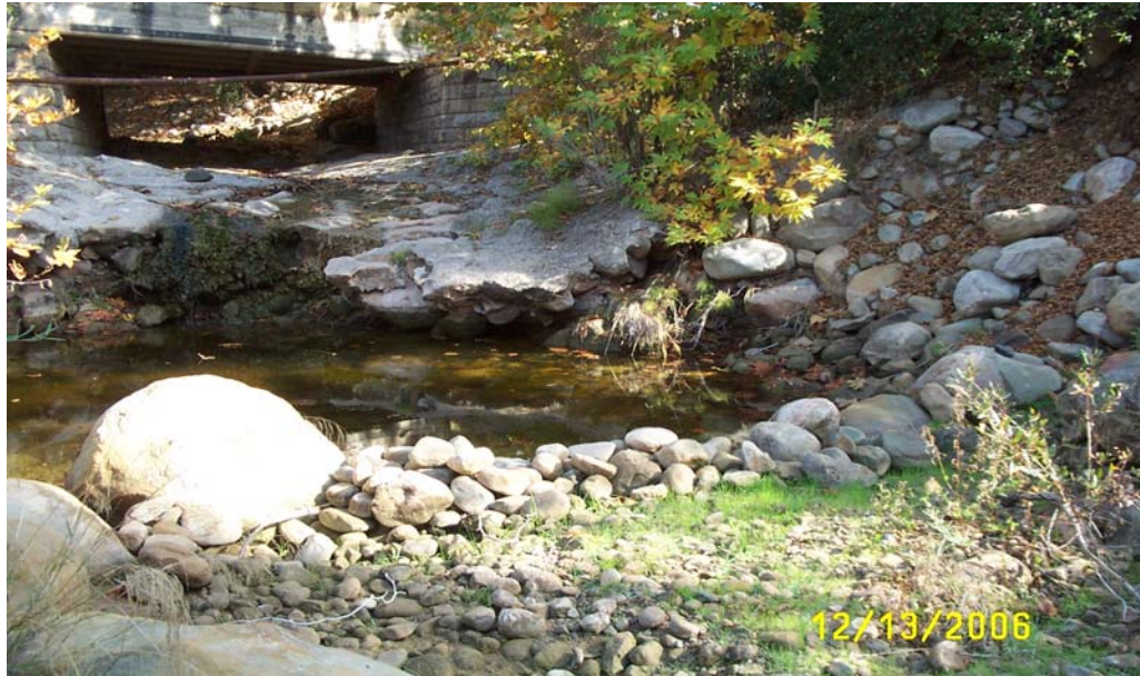
Arroyo Parida Creek and Bridge (12/13/2006), view upstream
