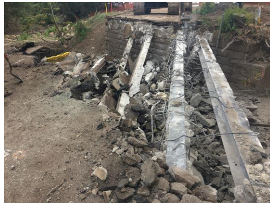
Photos of Arroyo Paredon Bridge Demolition on State Route 192 this morning.
