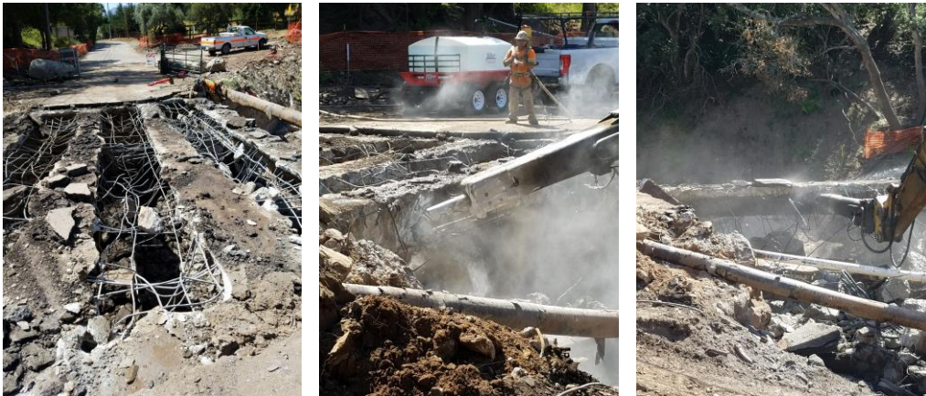
Photos of Toro Canyon Bridge Demolition on State Route 192 on May 14.
