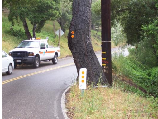
Mature oak tree to be removed on State Route 192 to improve sight distance for motorists.
