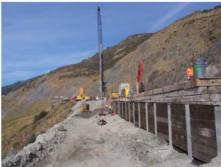
Retaining Wall north of Bridge—January 12, 2012
