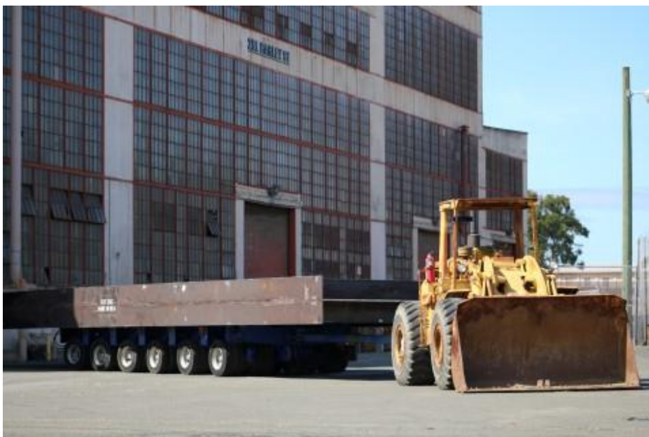
Completed girder leaving the plant.
