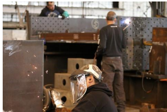
Steel girder in pre-stages of fabrication.
