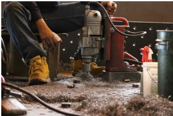
Photo of bolt hole drilling on steel girder.
