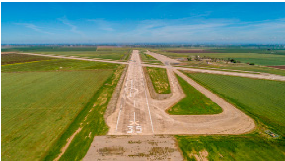
Crows Landing Industrial Business Park
