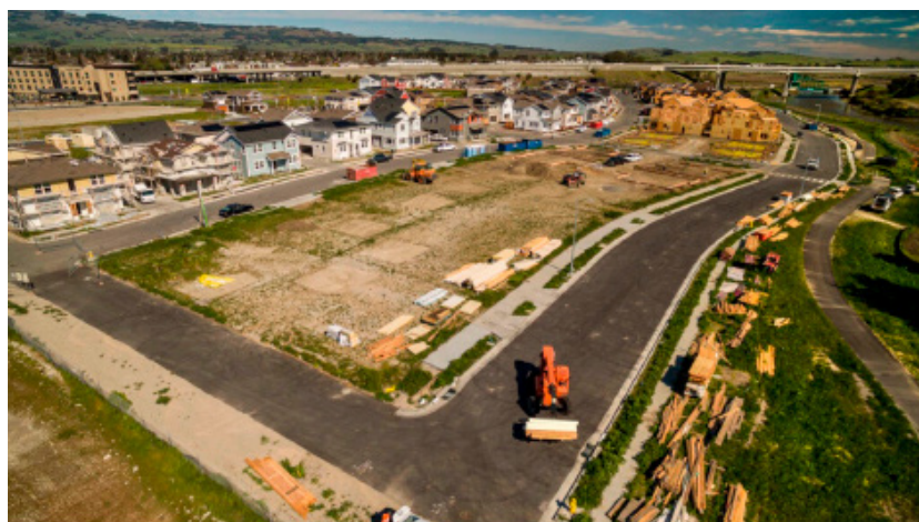
Riverfront in Petaluma Currently Under Construction
