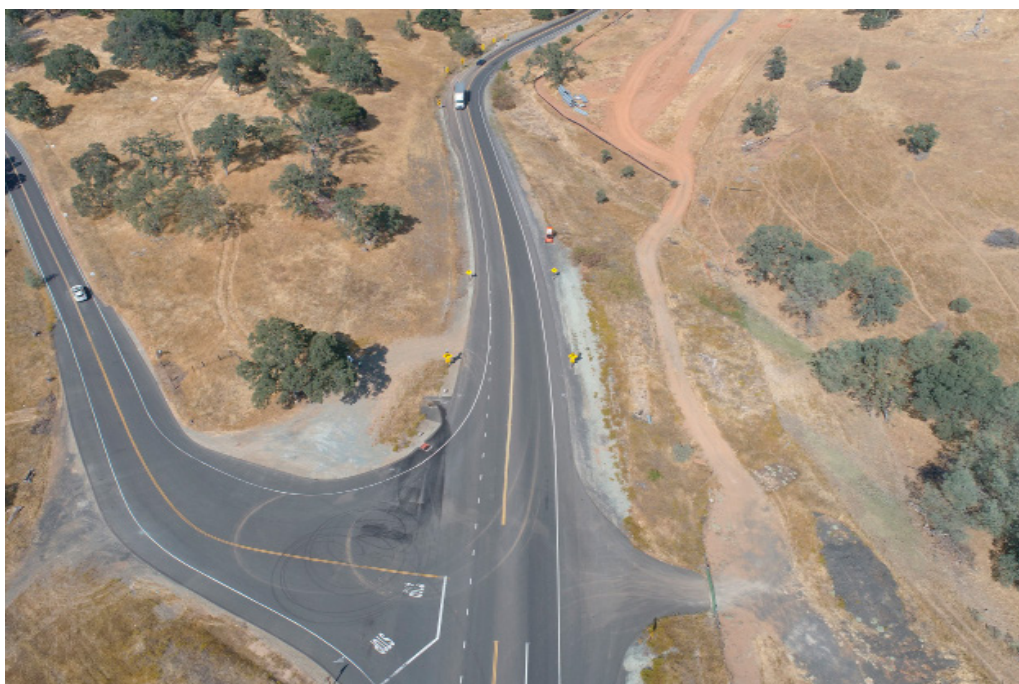
Wagon Trail Realignment Project
