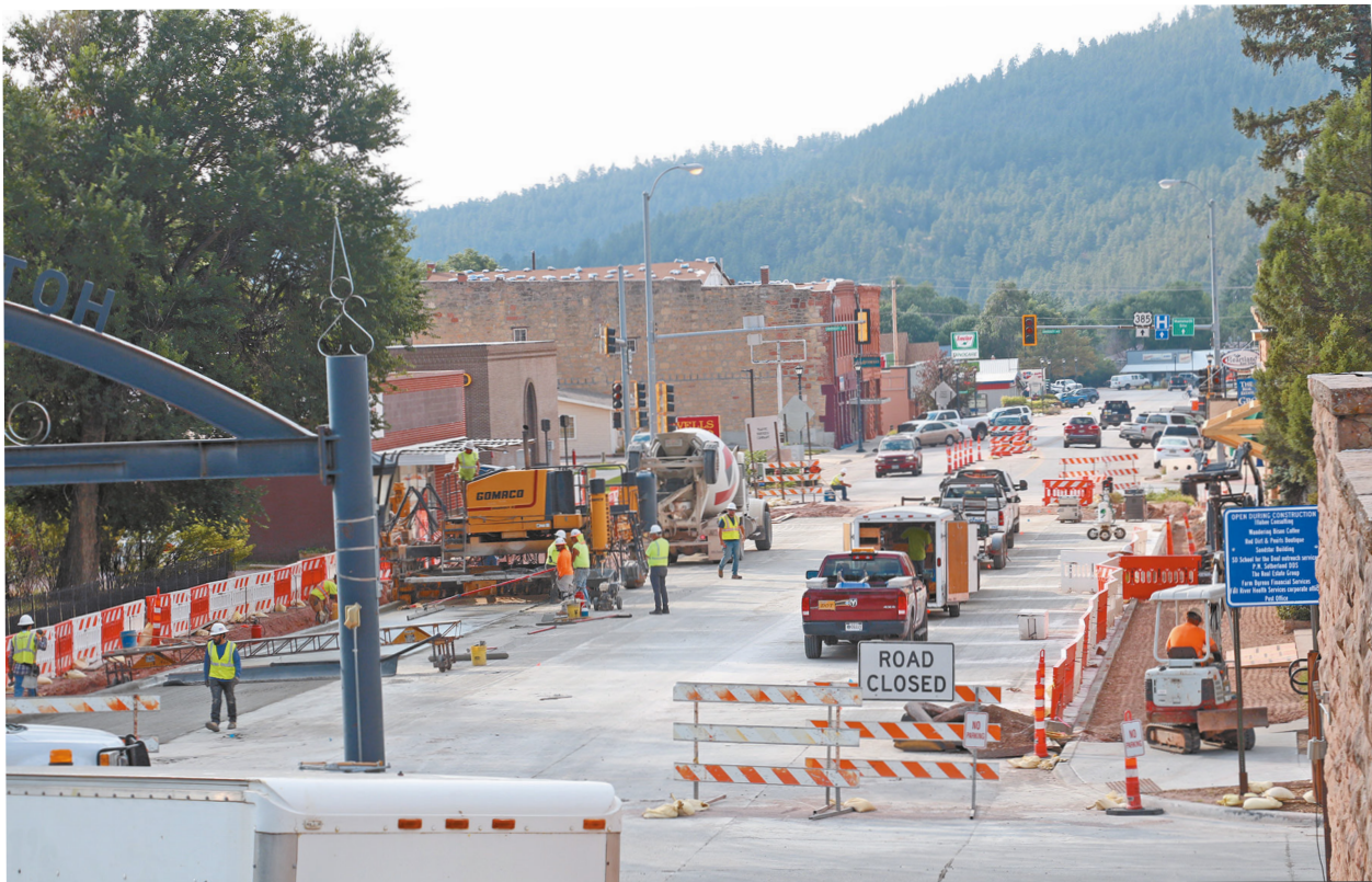
Hot Springs Road Under Construction
