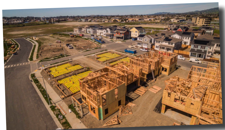
Riverfront in Petaluma Currently Under Construction
