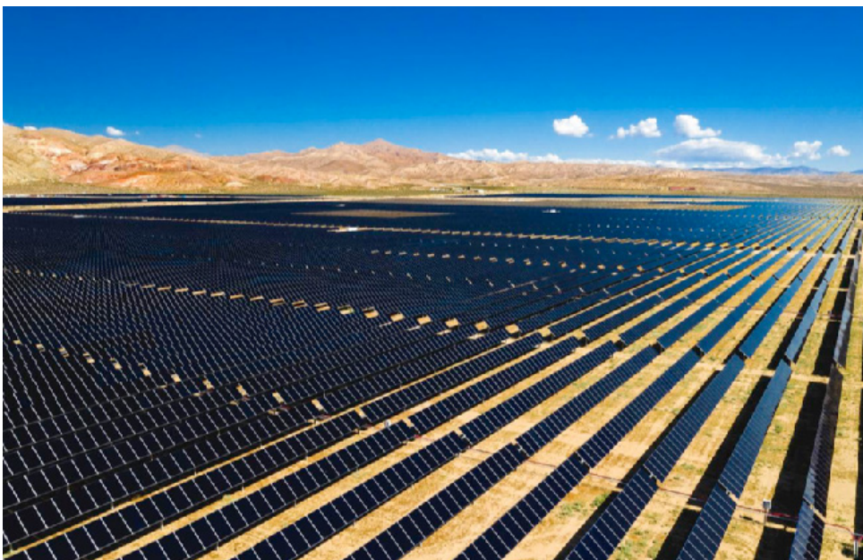
8minute Solar Energy’s 121-megawatt Solar Farm was completed in 2019 in Cantil. It was the first phase of a 1,500-acre project that began in 2015. The farm provides electricity to power more than 150,000 homes in the Los Angeles metro area.
