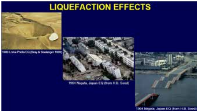
Figure 1: Examples of liquefaction effects. (Courtesy of John Bray, UCB)
