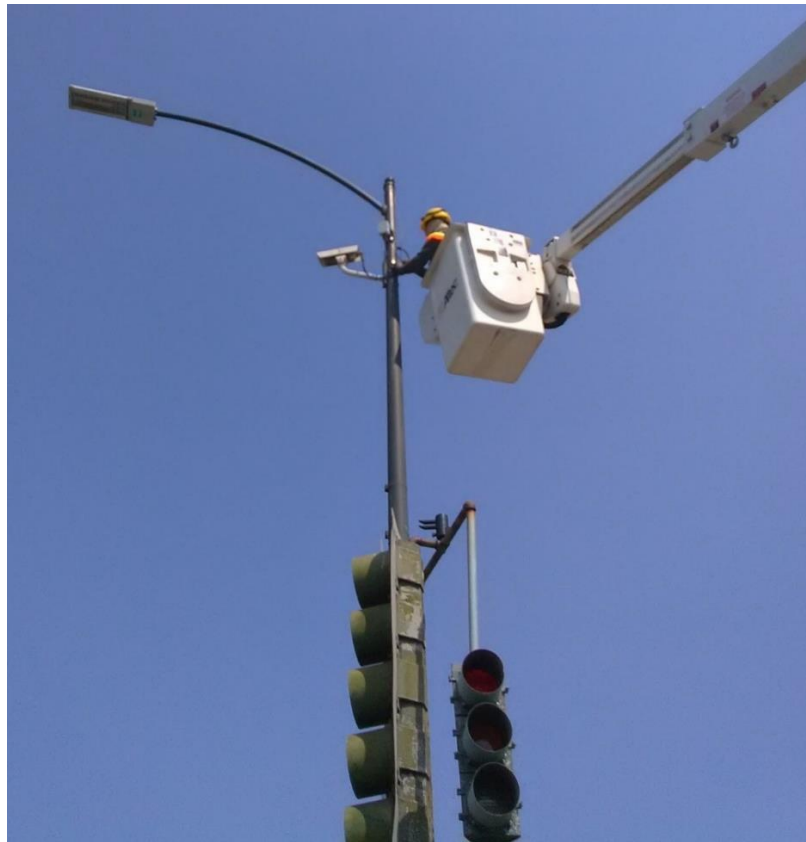
Figure 16 - mounting a Sensys SPP radio on the traffic signal standard
