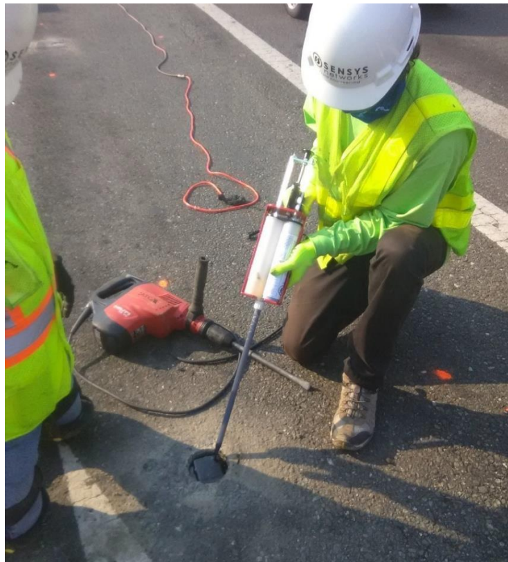
Figure 12 - Filling hole to road surface
