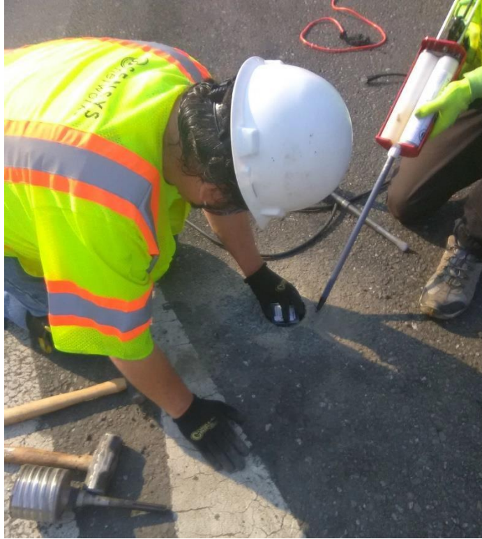
Figure 11 - Placing magnetometer
