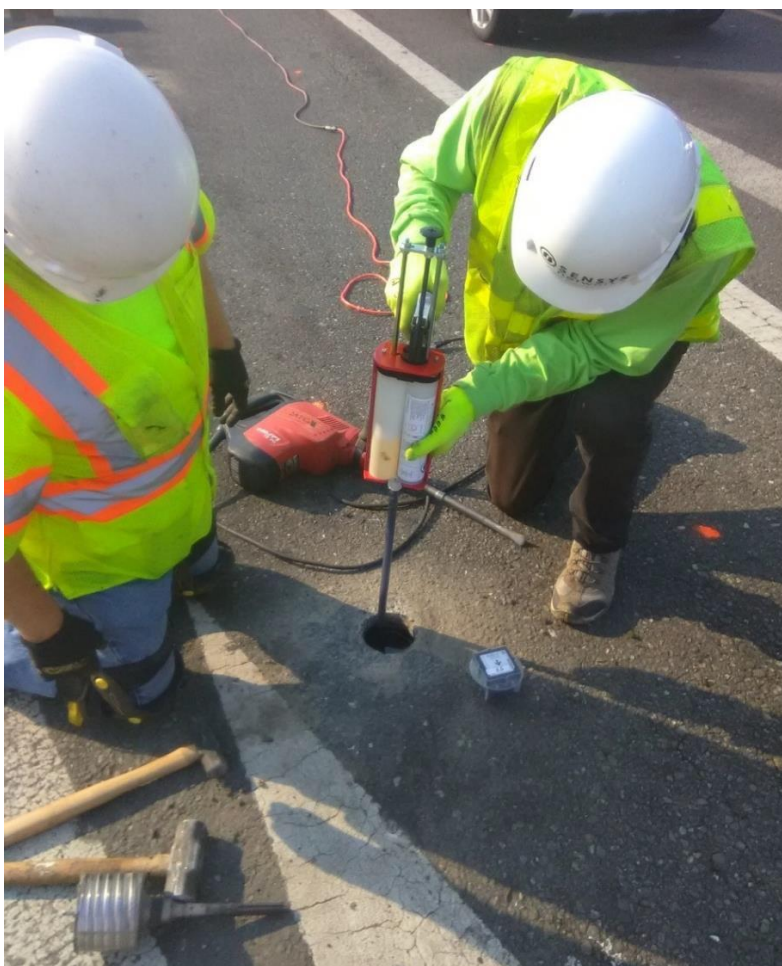
Figure 10 - Filling the bottom of the hole with epoxy
