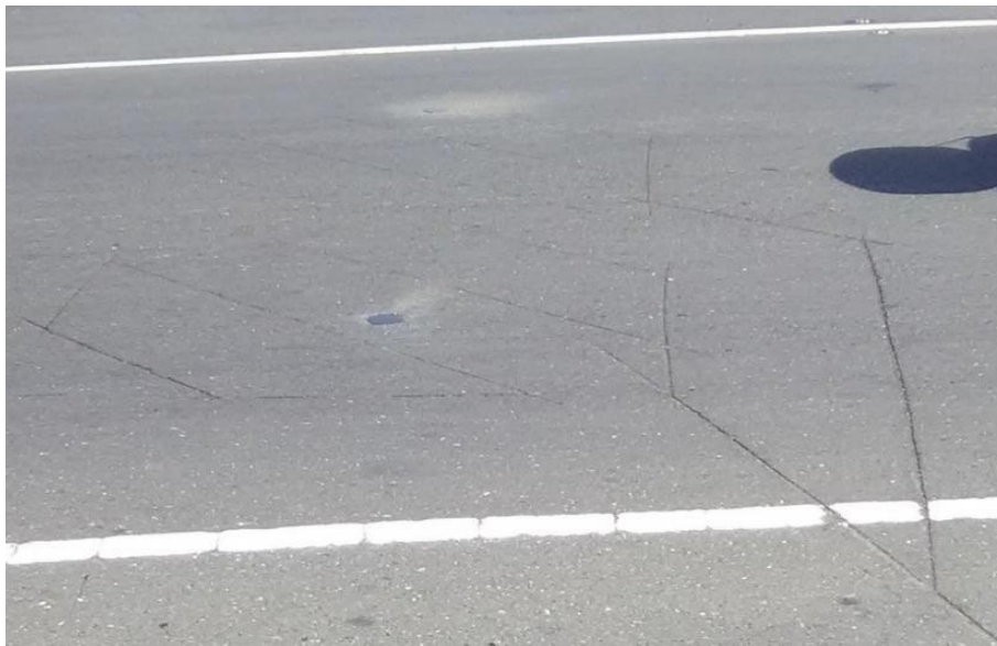
Figure 32 - two Sensys magnetometers installed abreast in unusually wide lane
