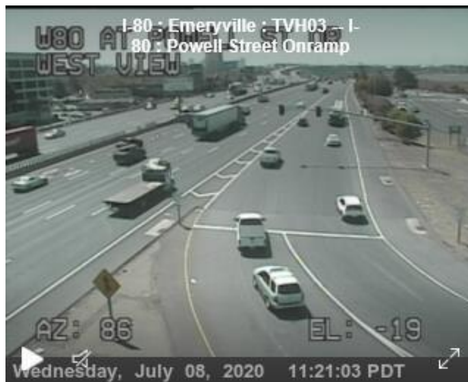
Figure 2 - Sensys detection zones at ramp meter location
