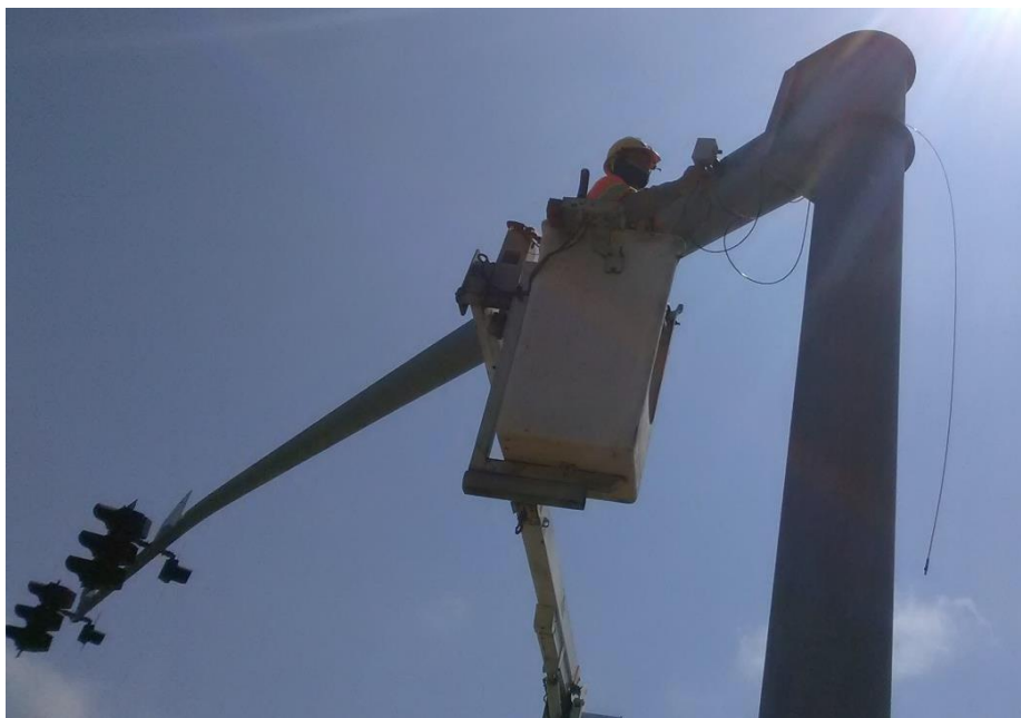
Figure 14 - mounting a Sensys SPP radio on the ramp meter standard
