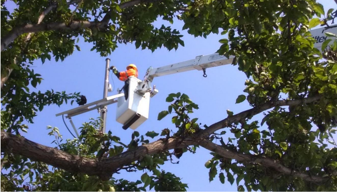
Figure 17 - mounting Sensys repeater on Trailblazer sign pole
