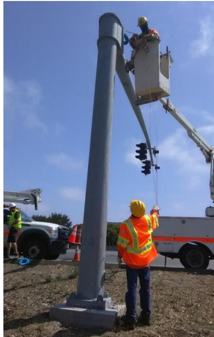
Figure 13 - Pulling Cat5e cable into ramp meter standard with fish tape
