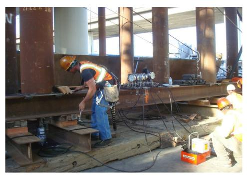
Figure 3-19. Jacking System Transferring Load to Temporary Support, San Francisco
