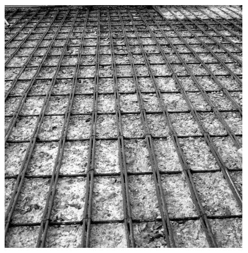
Figure 3-12. Hydroblasting for Partial Deck Removal
