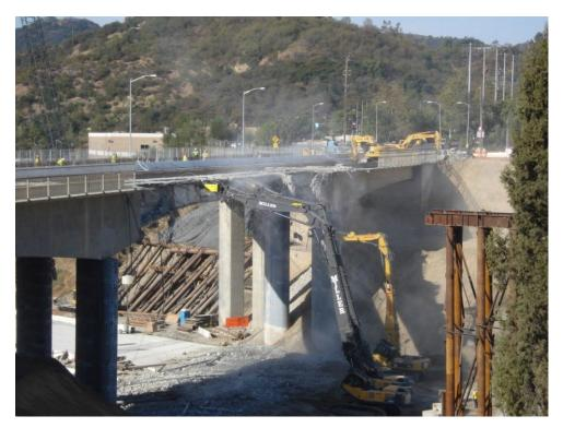
Figure 3-1. Long Reach Excavator at Mulholland Drive, Los Angeles
