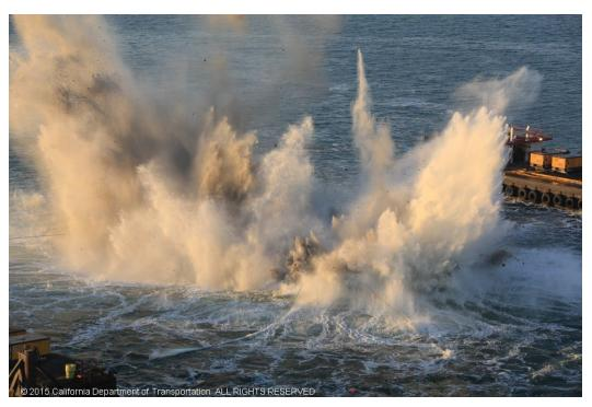
Figure 3-14. Explosive Demolition of a San Francisco-Oakland Bay Bridge Pier
