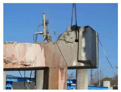
Figure 3-7. Diamond Wire Saw
