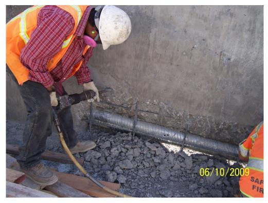
Figure 3-9. Handheld Pneumatic Hammer, Bear River
