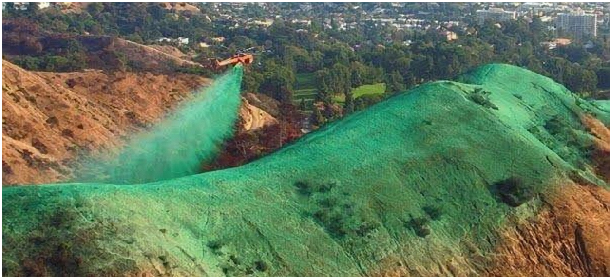
After a wildfire, slopes are vulnerable to mudslides during and after rain. To mitigate risks to transportation infrastructure, Caltrans uses hydroseeding by helicopter to reseed burned slopes. (credit: Caltrans)
