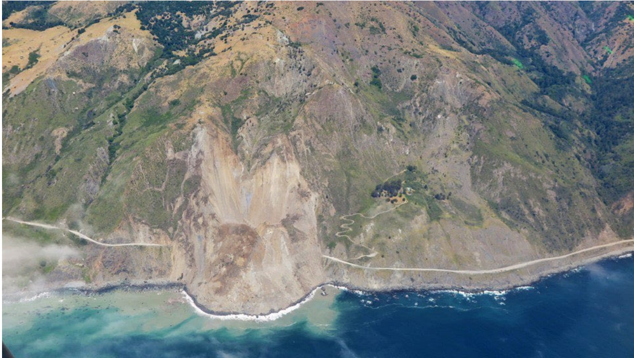
The Mud Creek Slide in Caltrans District 5 demonstrates how this stretch of Highway 1 is vulnerable to changing rainfall patterns. The slide occurred days after heavy rainfall during one of the wettest winters in a century for the area. (credit: Caltrans District 5)
