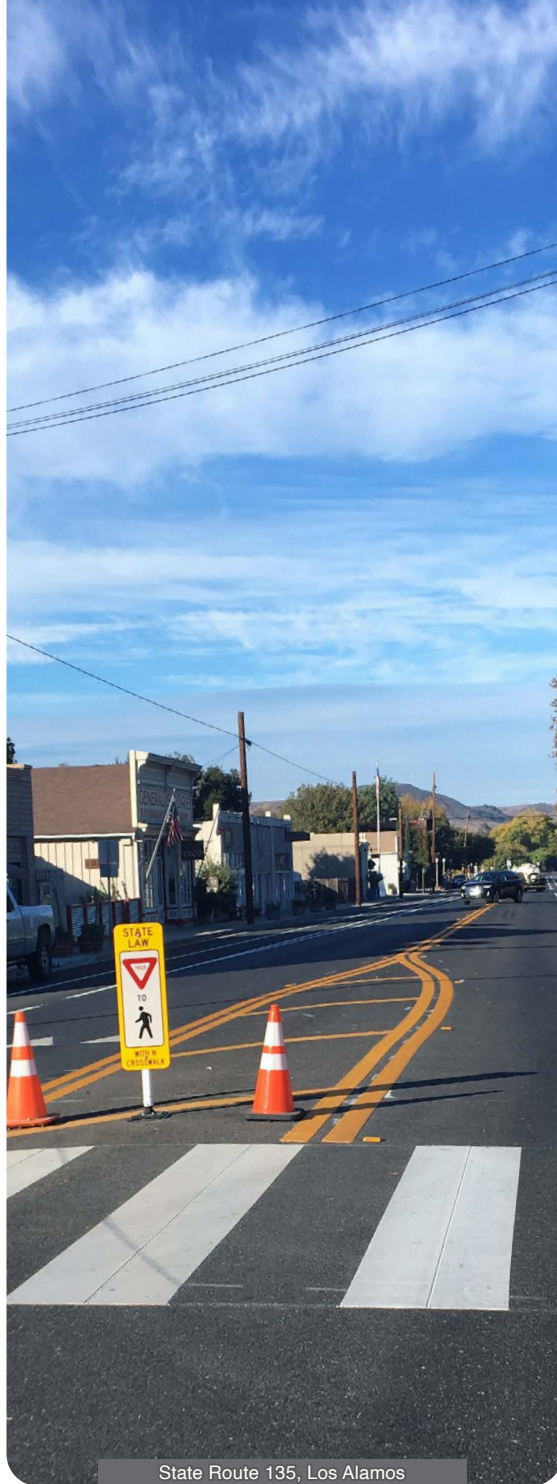
State Route 135, Los Alamos
