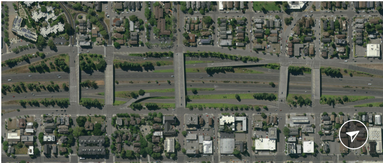
Photo 3: Current aerial view of I-980 separating West Oakland (top) from Downtown Oakland (bottom). The Vision 980 Study will seek alternatives to reconnect these two communities.
