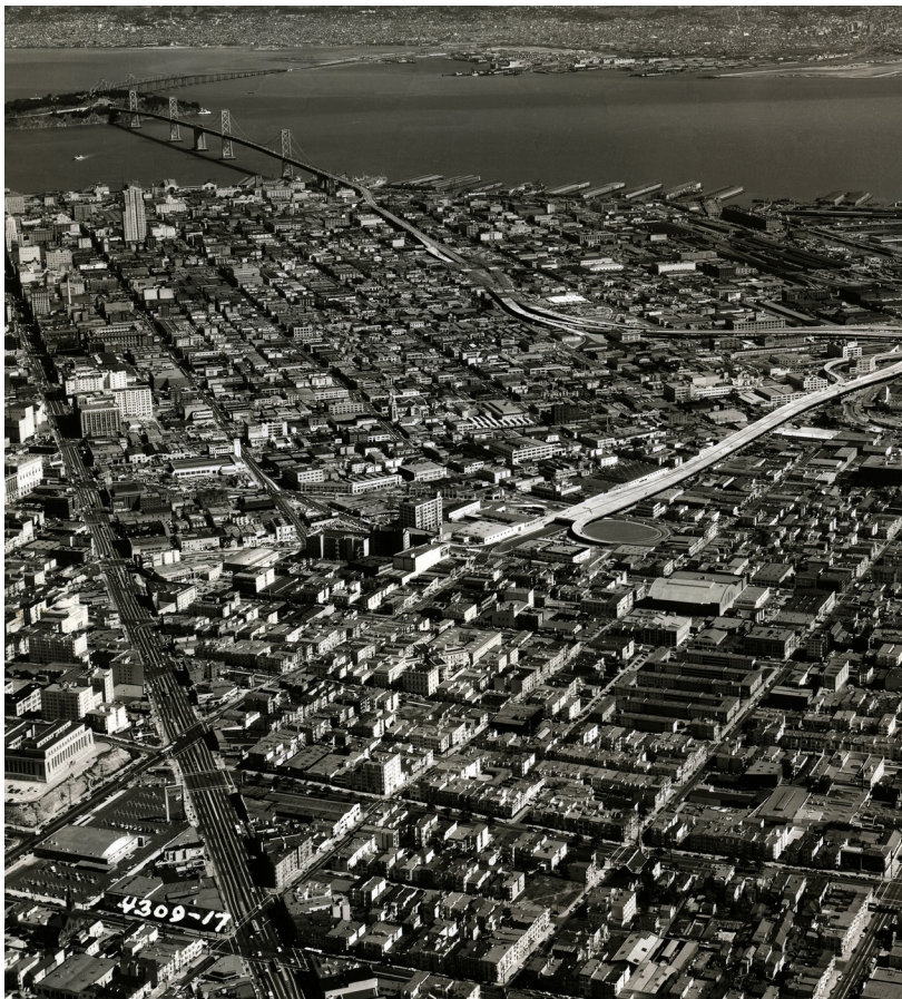
Photo 4: Aerial view of the Central Freeway, where it ended at South Van Ness Avenue in the mid-20th century.
