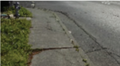
SIDEWALKS IN FAIR OR POOR CONDITION SHS segments with sidewalks in fair or poor condition, as determined by Caltrans staff.
