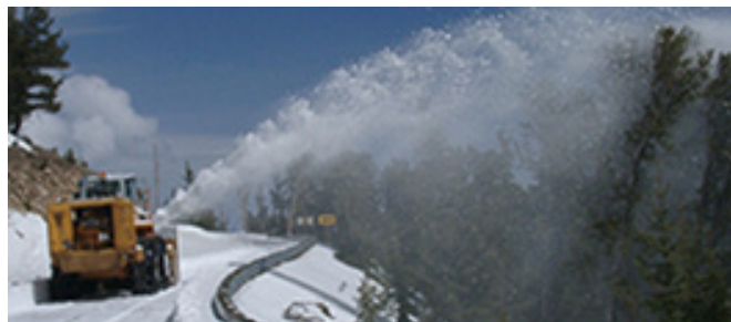
Image 1: Rotary blower removing snow from roadway
