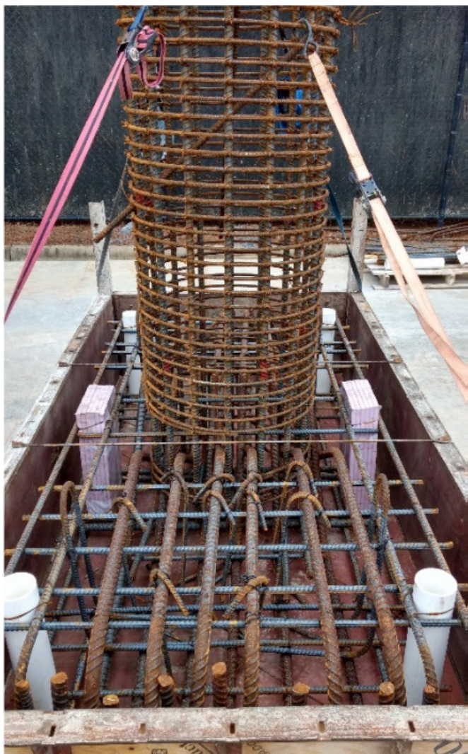
FIGURE 1: column and footing rebar
