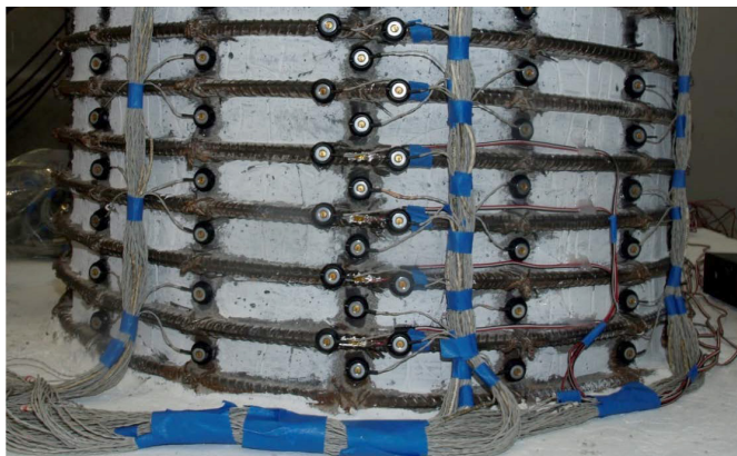
FIGURE 4: Optotrak markers in block-out regional damage state
