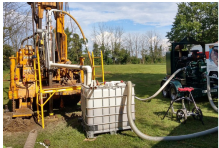
Image 2: The ISTD equipment assembled for field test 3
