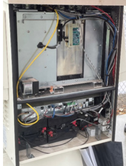
Image 3: Hydrogen Fuel Cell – Image Source: Caltrans
